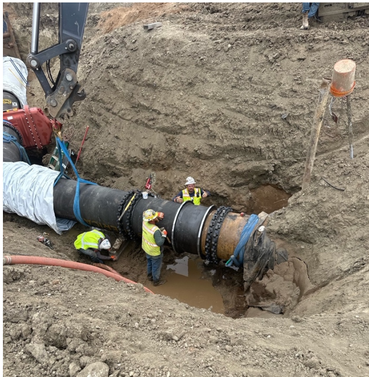
Photo 2: Contract 2-1E – Installation of Discharge Pipeline on August 21, 2024
