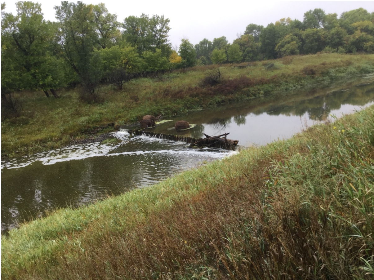
EASTSIDE ESTATES DAM 1 – DWR PHOTO 2019
