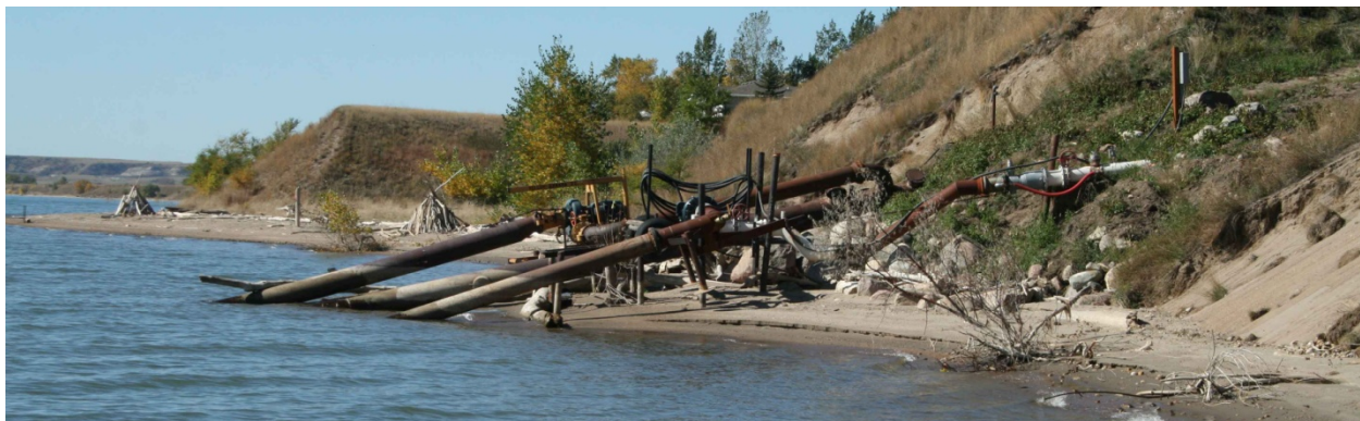
Figure 6 Existing Water Intake East of Whitetail Bay
