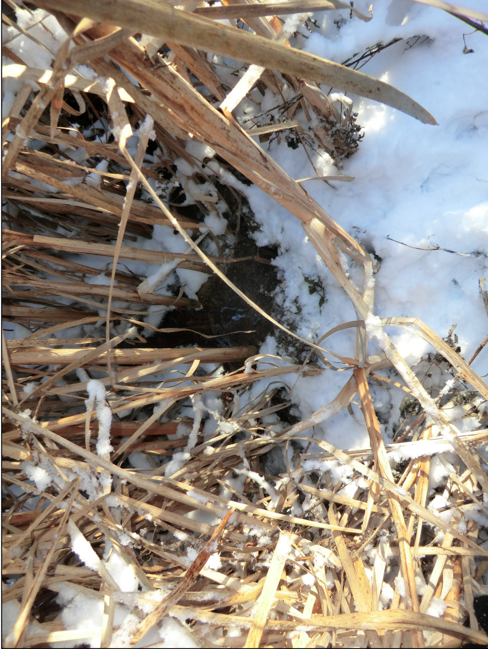
Figure 5. Seep on the right embankment east of the large tree.
