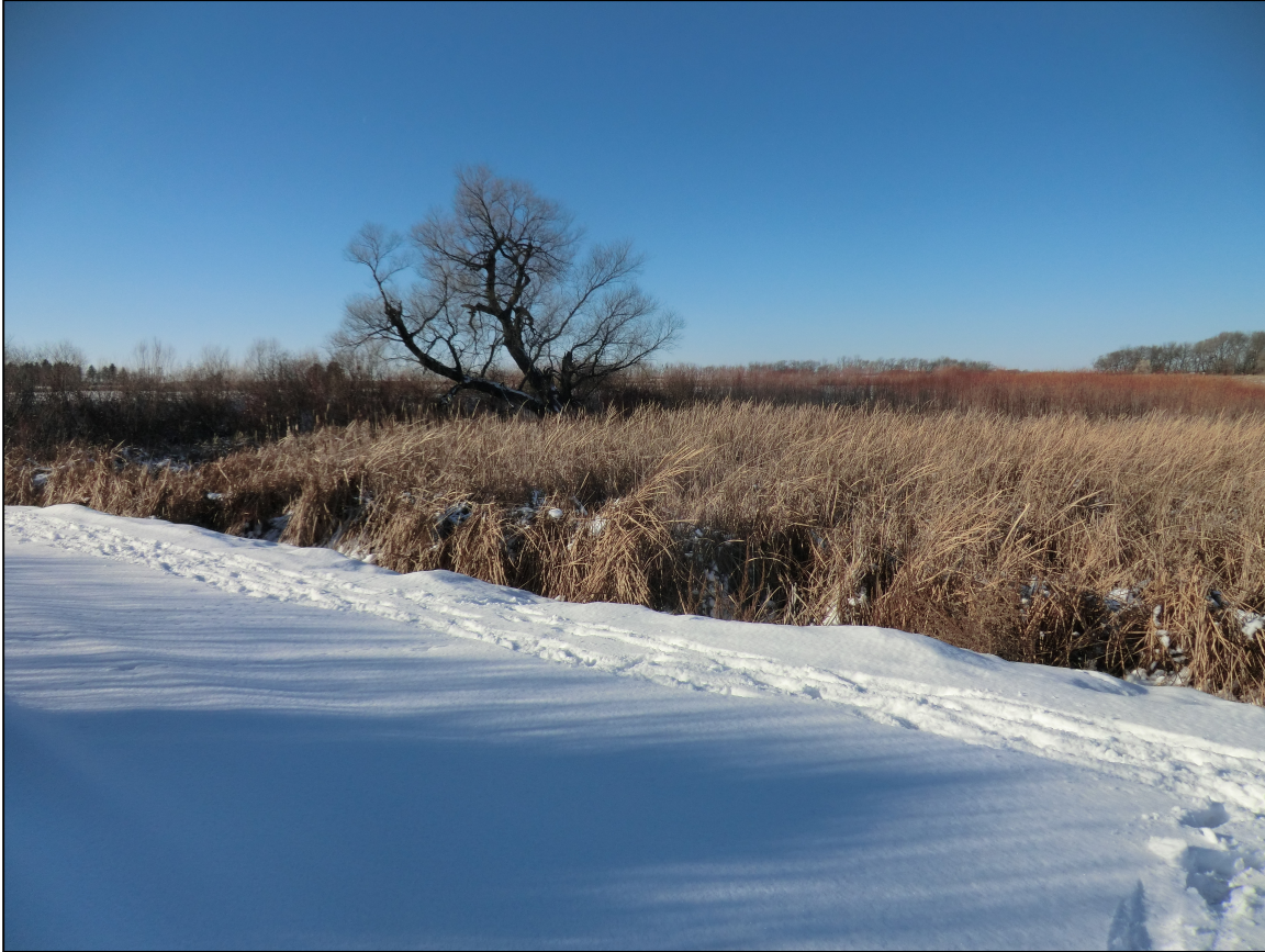
Figure 3. Silver Lake Dam, right embankment (photograph taken from downstream side).
