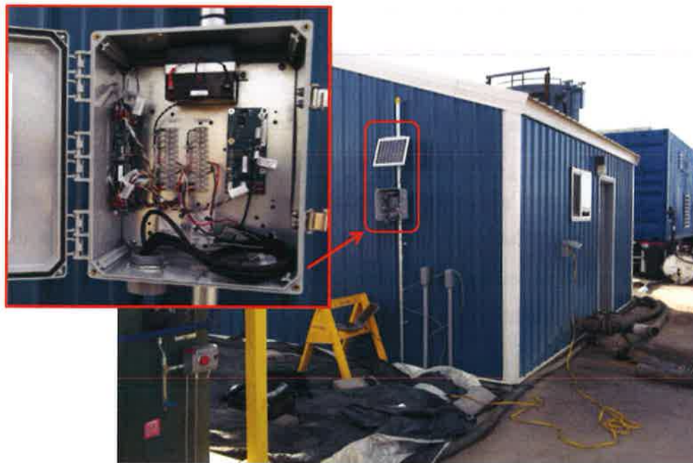
Figure 2. Installation of McCrometer Telemetry at Timber Creek Depot operated by Mike Ames.
