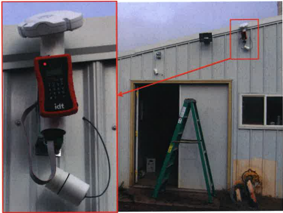
Figure 4. Installation of IDT Telemetry at the Schaper Water Depot owned by Jim Schaper. Exterior view of the telemetry system, with the hand-held calibration system.
