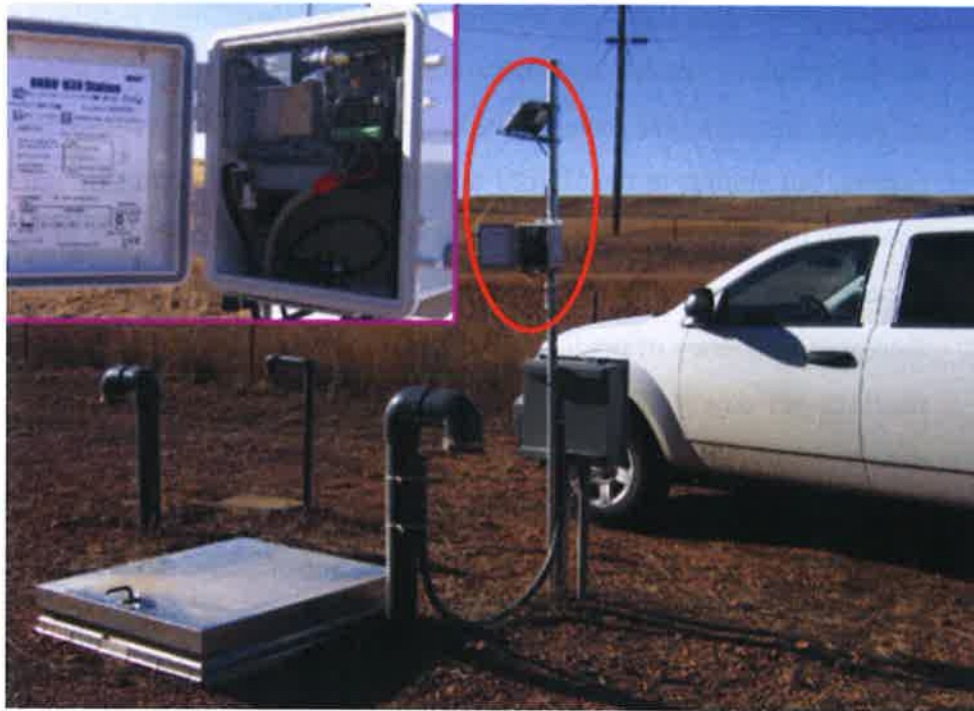
Figure 1. Installation of On-Set Computer HOBO Data Logger at the Dodge Depot operated by SWWA
