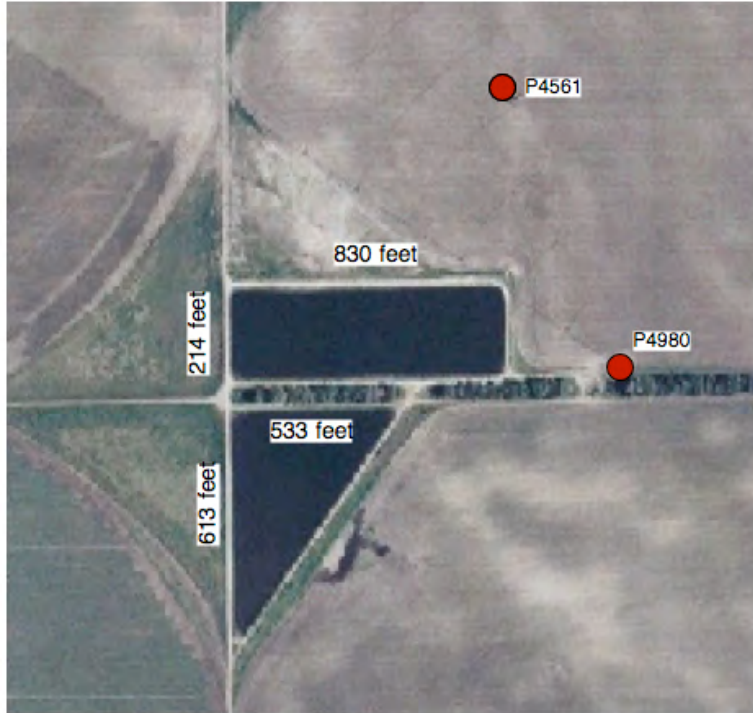
Figure 13. ARR recharge basins and local recovery wells (red).
