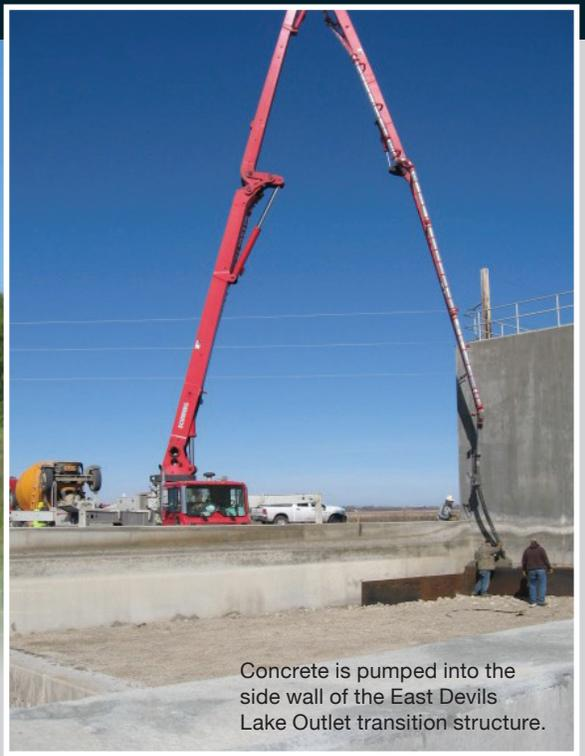
Concrete is pumped into the side wall of the East Devils Lake Outlet transition structure.
