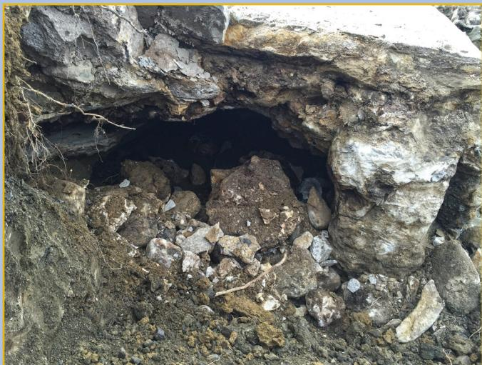
Water flowed underneath Tolna dam and caused internal erosion that can be seen here.
