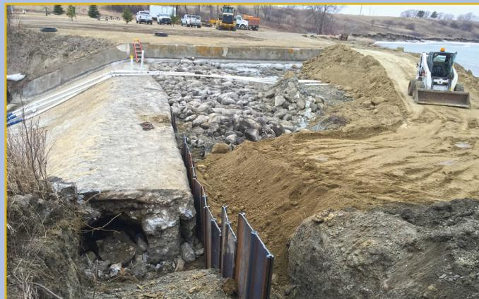
Repairs being made to Tolna Dam. The reservoir was drawn down and a cofferdam was constructed to allow access to areas needing repairs.
