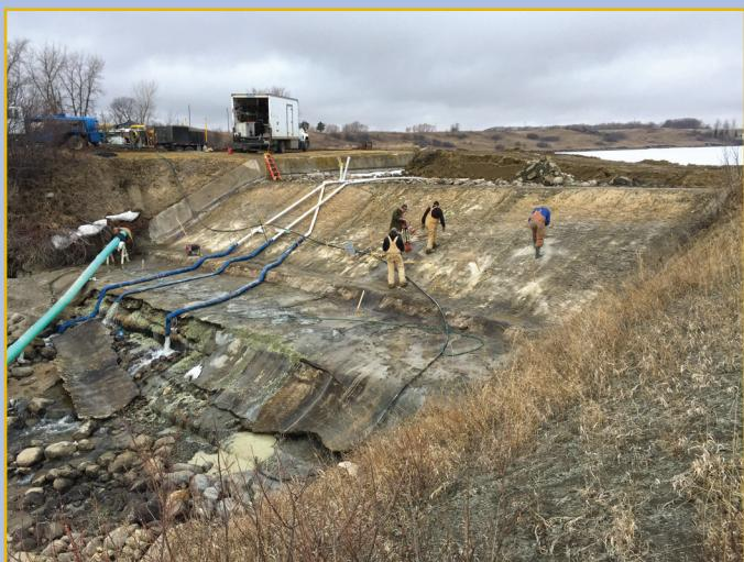
Members of the construction crew searching for voids underneath the spillway. When voids were found, grout was pumped into the structure to fill them.
