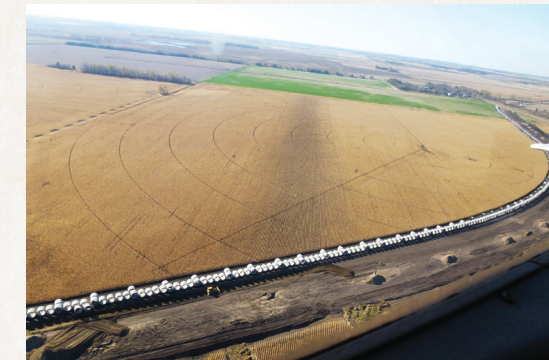
An aerial view of 96” pipe being staged for installation along the route of the East Devils Lake Outlet in 2011.
