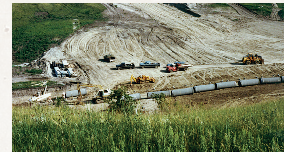
Construction on Dead Colt Creek in 1983.
