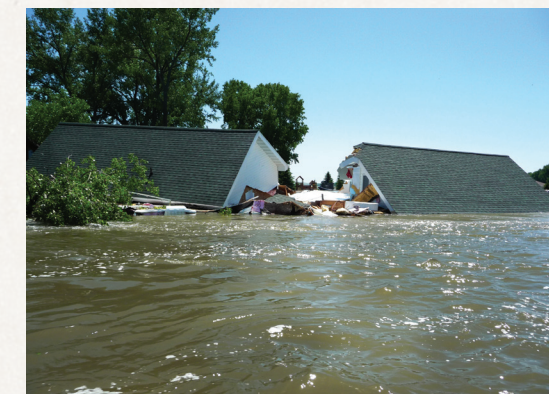
A house collapses into the Missouri River due to bank erosion during the record 2011 flood.
