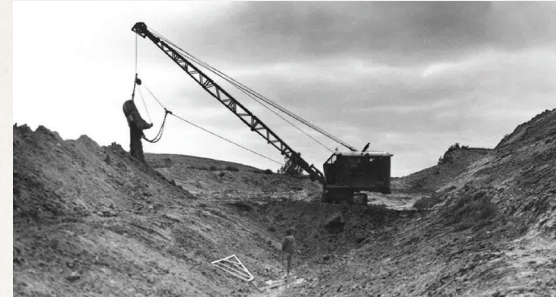
A drag-line excavating the main canal for the Buford-Trenton irrigation district in Williams County, ND.
