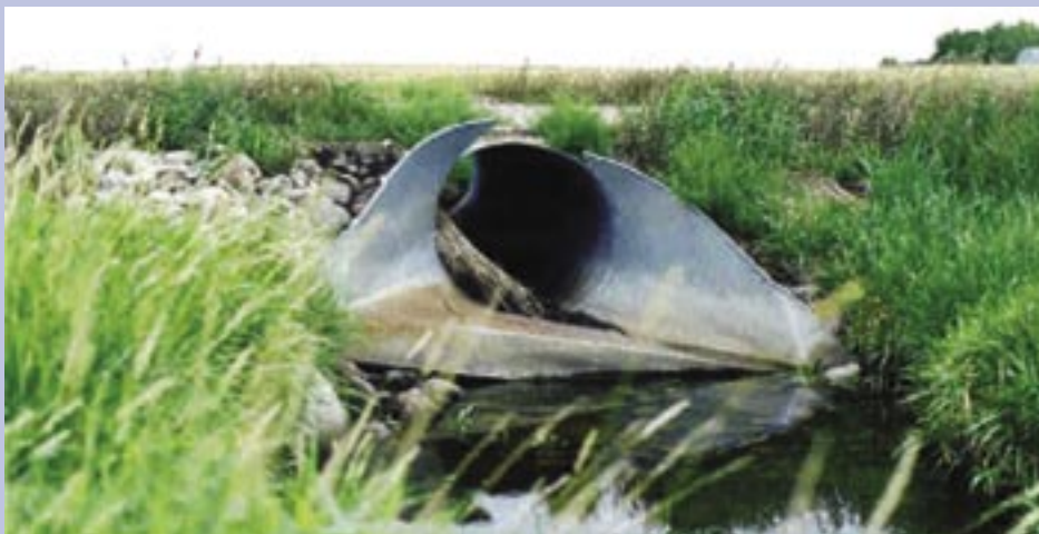
A culvert in Calio Coulee in the Devils Lake basin.
