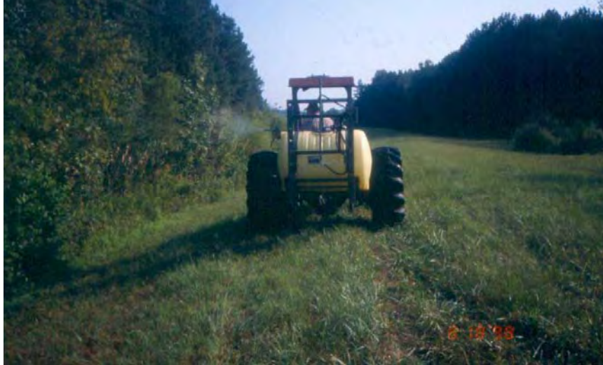
Figure 5f. Tractor spraying application on dam.
