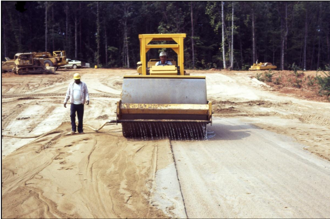
Figure 7-24. Compacting a joint between two zones by a vibratory roller.
