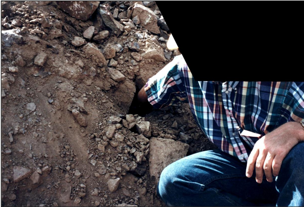
Figure 6-6. Open work present in the right abutment foundation of Ochoco Dam. The abutment consists of landslide debris.
