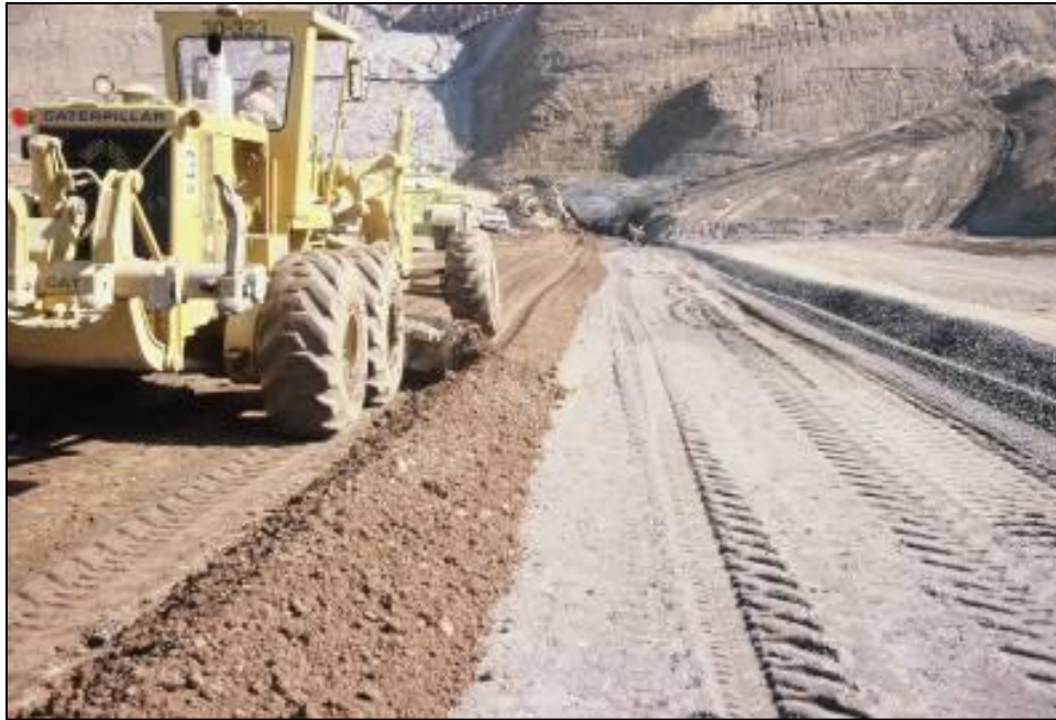
Figure 7-3. Windrowing impervious material adjacent to a filter/drain.
