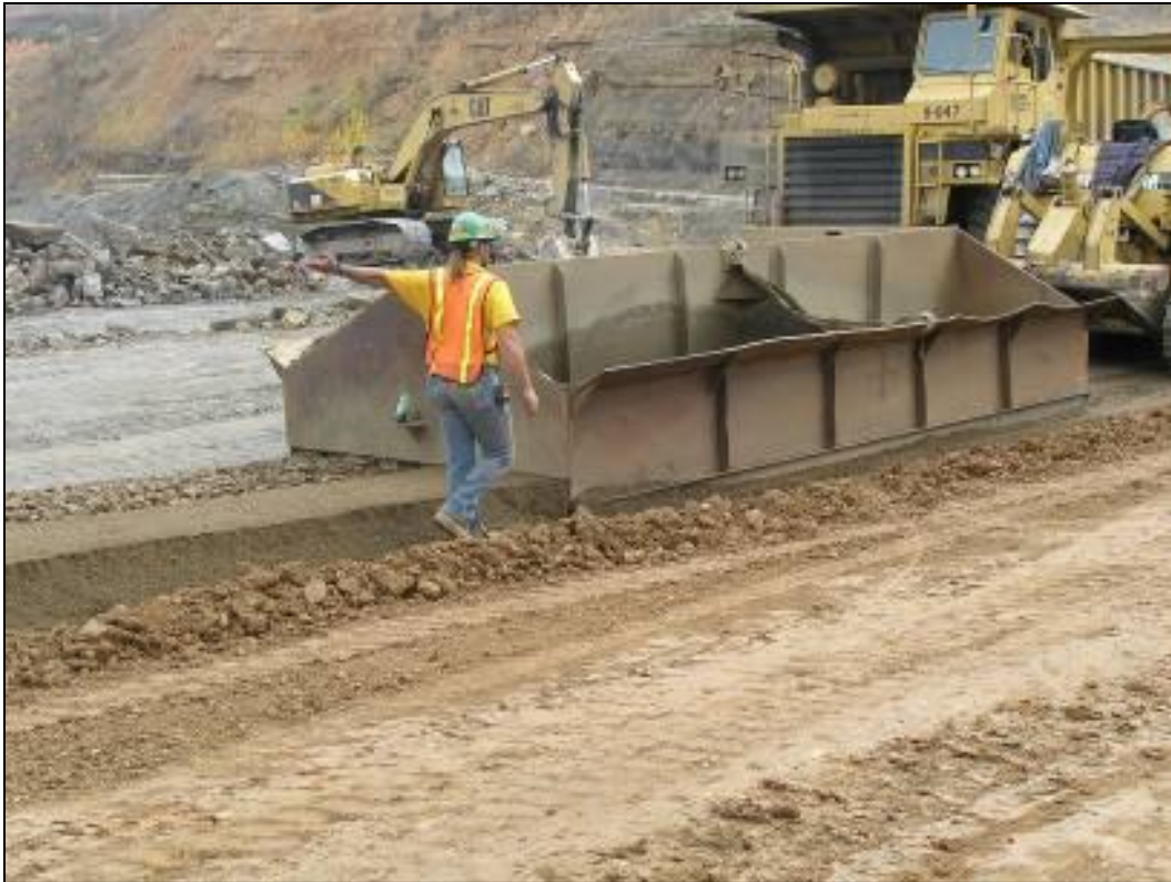
Figure 7-17. Towing spreader box.
