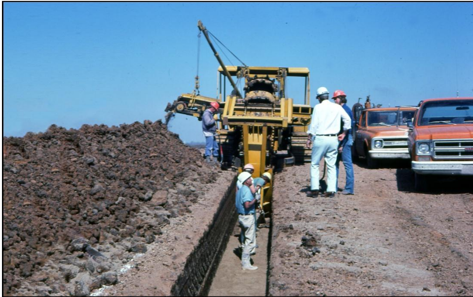
Figure 7-5. Trenching method – excavating trench.
