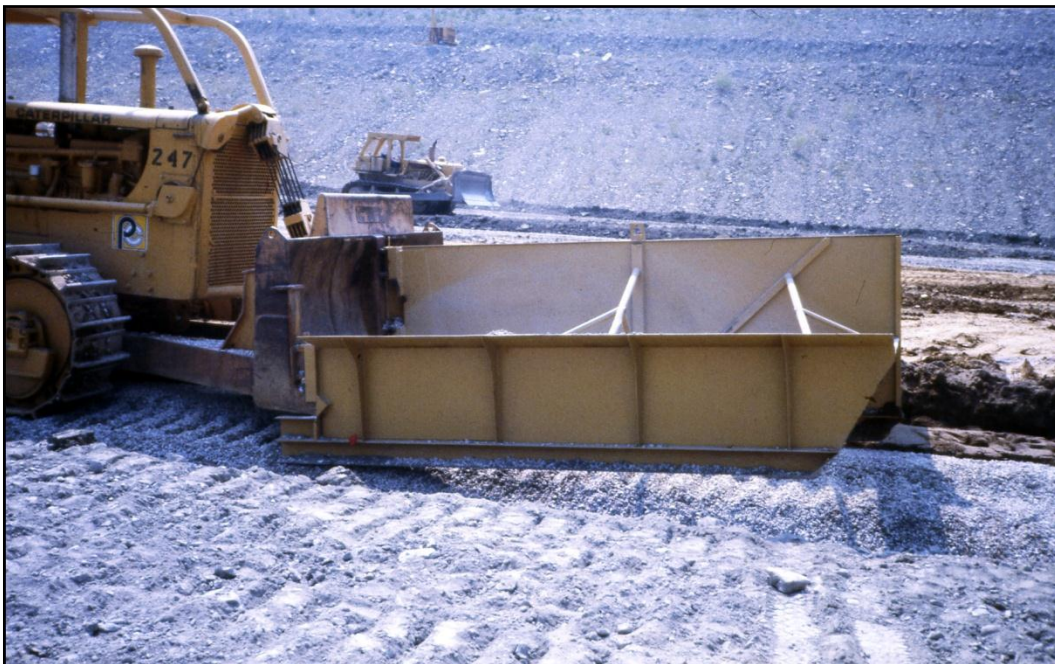
Figure 7-18. Double-bin spreader box fitted to dozer – side view.
