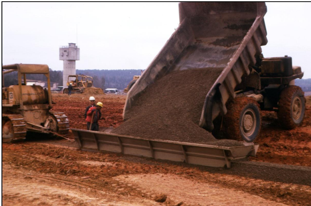
Figure 7-16. Dumping into spreader box.
