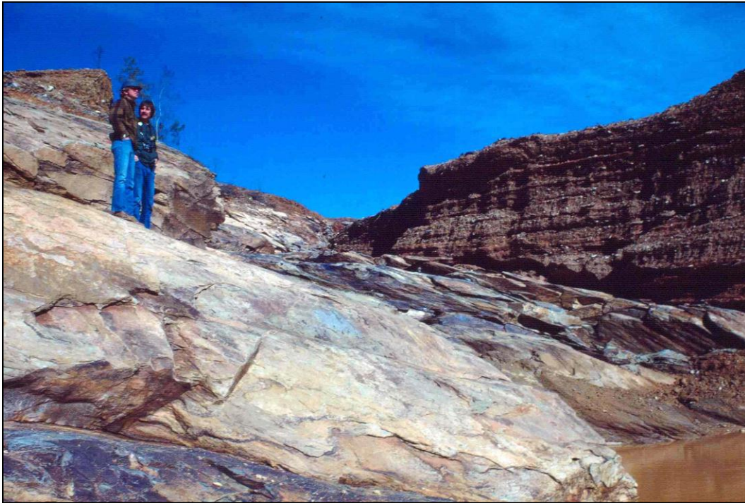
Figure E-5. Closeup of right abutment viewed upstream. Bedrock was cleaned by erosion from overtopping flow. Embankment is in top right of photograph.
