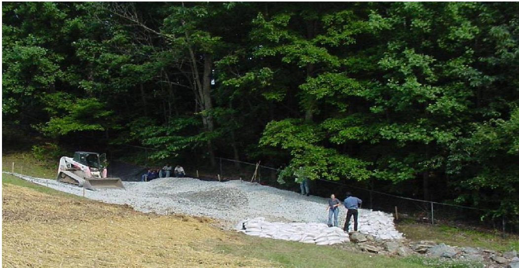
Figure L-26-2. Gravel drain being placed over seepage area.
