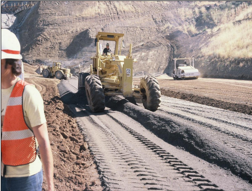
Figure 7-13. Spreading sand filter material.
