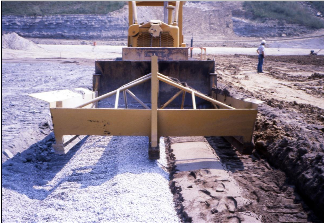
Figure 7-19. Double-bin spreader box fitted to dozer - front view.
