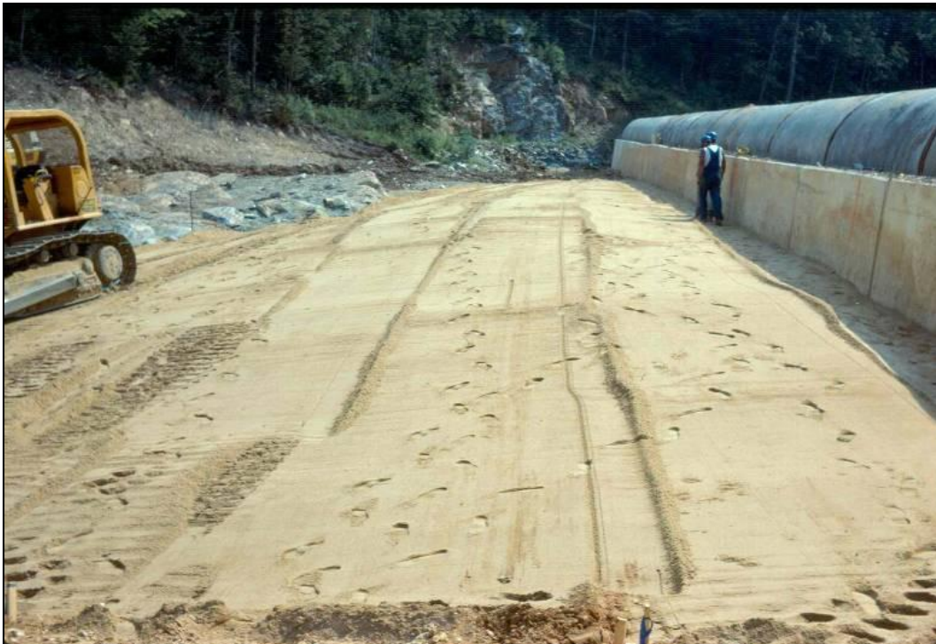
Figure 2-11. Fine filter placed over gravel blanket drain shown in Figure 2-10. (Photo courtesy of NRCS, Alabama.)
