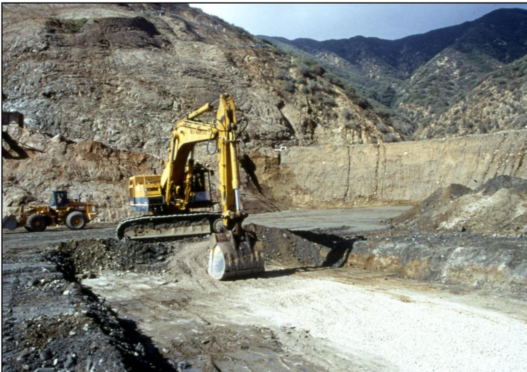
Figure 7-27. Excavation of filter material under equipment crossing.
