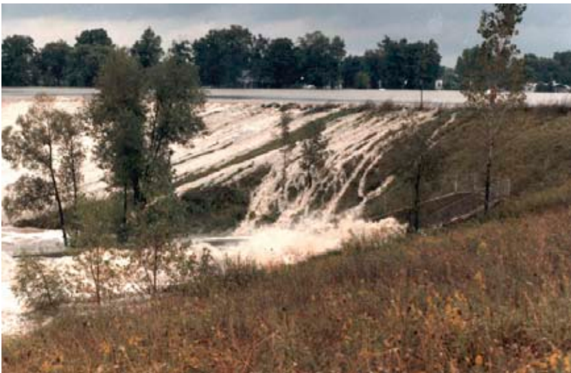
Overtopping can fail an earthen dam.
