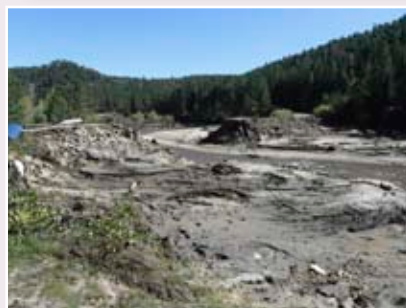
Above: Upgraded dam with spillway operating correctly.
