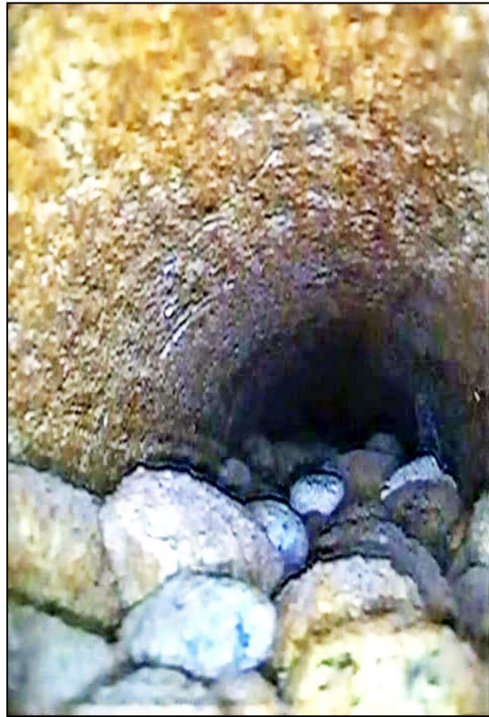
Figure A-112. —Typical condition of Underdrain Nos. 2 and 3 downstream of the second bend, where camera could no longer be advanced.
