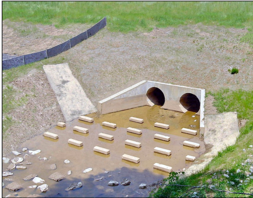
Figure 57.—Basin utilizing staggered rows of baffles.
