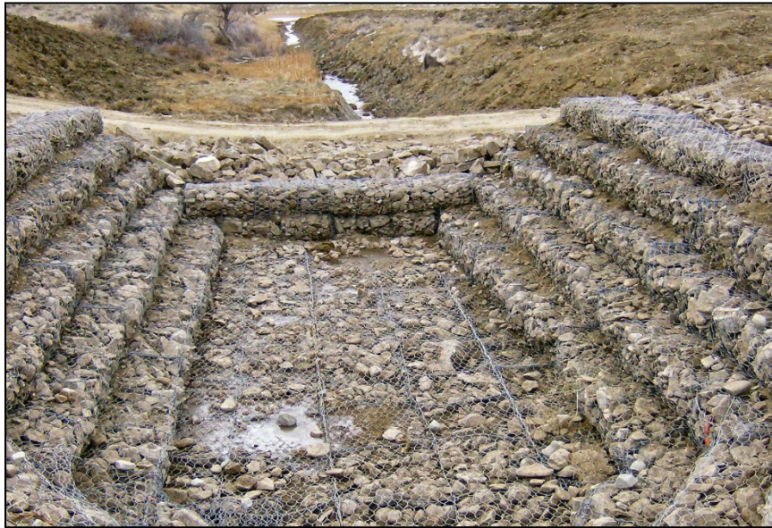
Figure 127. —Gabion-lined basin. The earthen basin was used to facilitate construction access and has been removed.
