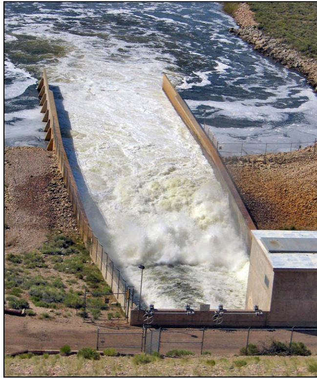
Figure 2. —A hydraulic jump occurring in an outlet works energy dissipator.
