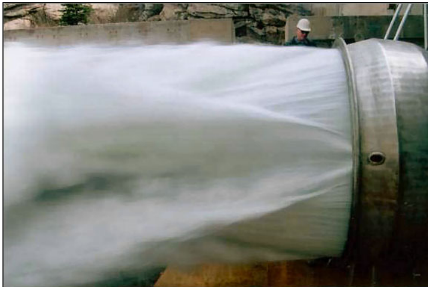
Figure 81. —48-inch diameter hooded fixed-cone valve discharge. Photo courtesy of URS Corporation and Denver Water Board.
