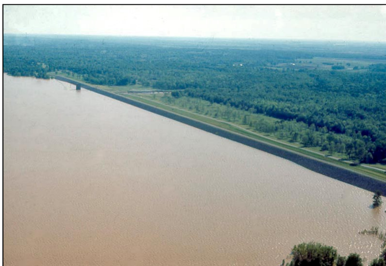
Figure A-6. —Aerial view of the upstream face of Arkabutla Dam.
