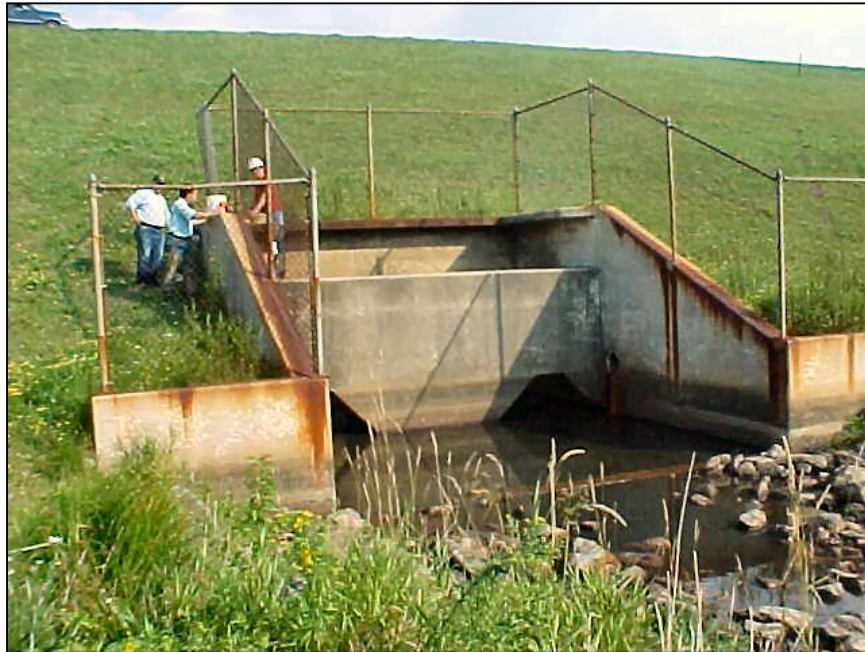
Figure 144. —A periodic inspection being performed at an impact basin.
