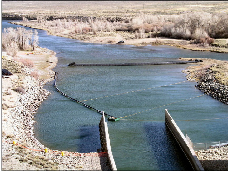
Figure 167. —A polyethylene baffled bladder dam is being placed downstream from a stilling basin. The dam is 250 feet long by 19 feet wide by 8 feet high. The dam weighs 2,600 pounds (dry). Two 3-inch pumps (8 hp) and two 3-inch pumps (4.5 hp) were used to fill the dam with 150,000 gallons of water. The dam took about four hours to deploy (watering up and rolling out the dam). Upon removal, the dam took 2 hours of dewatering and 2½ hours to roll up and remove. Removal of the dam required the rental and use of two track-hoes for rolling up the dam on a log.
