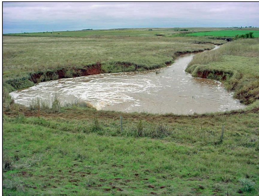
Figure 58. —Unlined plunge basin (view is looking downstream). This basin has been allowed to scour over time.
