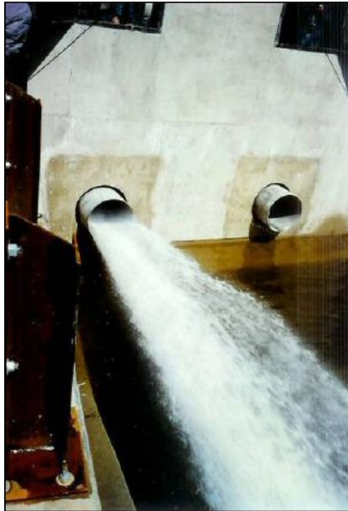
Figure 98. —Jet-flow gate at partial opening. Photo courtesy of URS Corporation.
