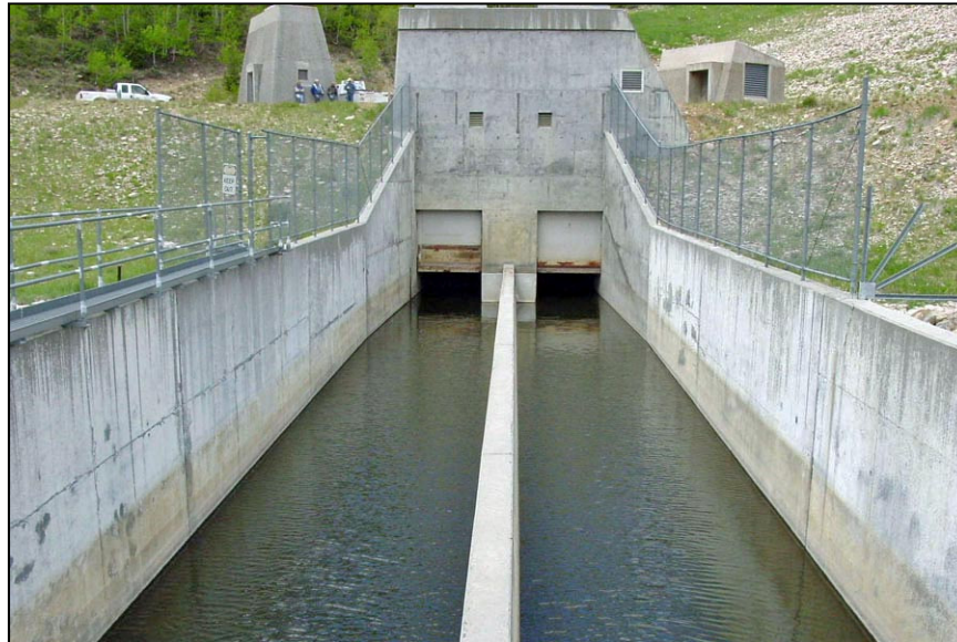
Figure 25.—Splitter wall separating discharge from two conduits.
