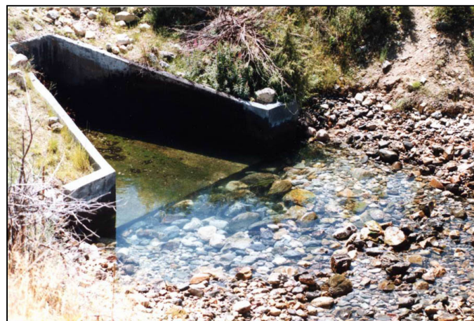
(c) Minor scour exists downstream from the structure after sustained discharge of 270 \text{ ft}^3/\text{s} .
