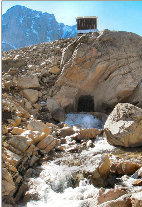
Figure 4. —If the downstream formation consists of competent rock where the potential for erosion is negligible, an energy dissipator may not be required.
