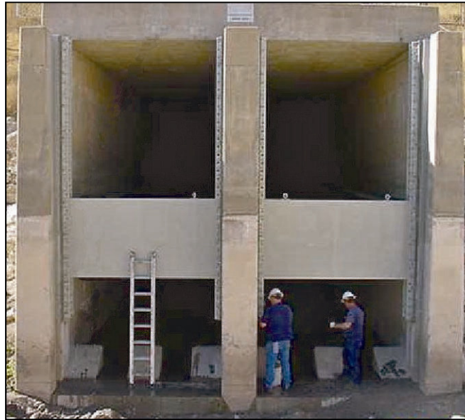
Figure 31. —Flow deflectors being installed at the downstream end of a stilling basin.
