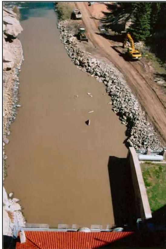
Figure 83. —A 48-inch diameter hooded fixed-cone valve. Note erosion of riprap in downstream channel. Photo courtesy of URS Corporation and Denver Water Board.
