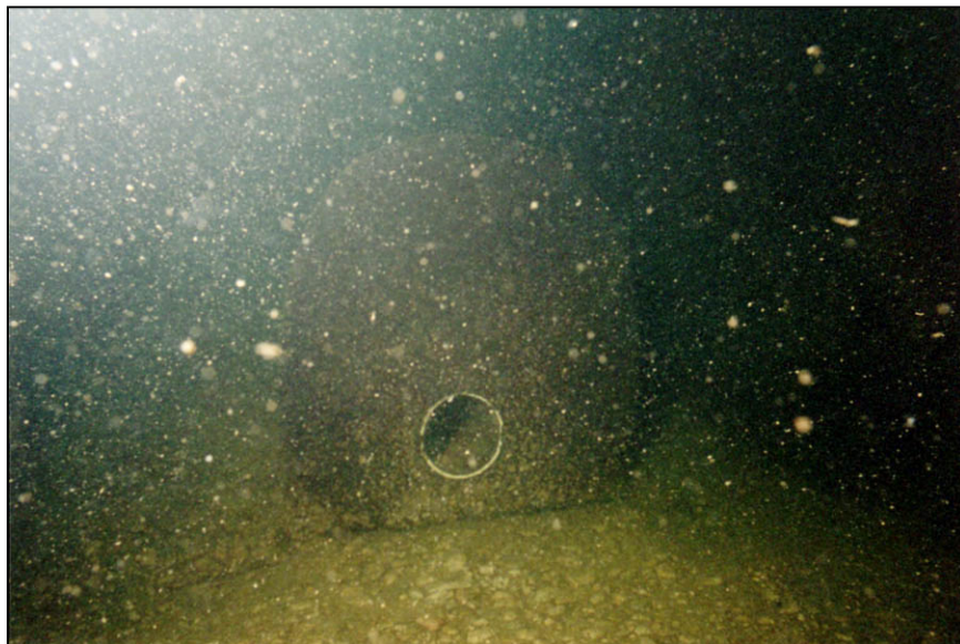
Figure A-106. —Typical condition of downstream face of outlet works stilling basin chute block and 6-inch diameter PVC drain outfall.
