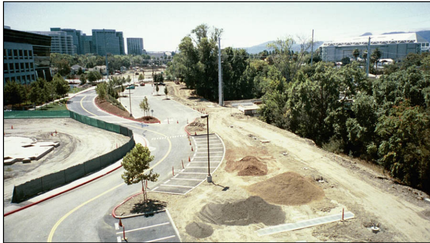
Figure A-29.—Culvert Under Sobrato Business Park.
