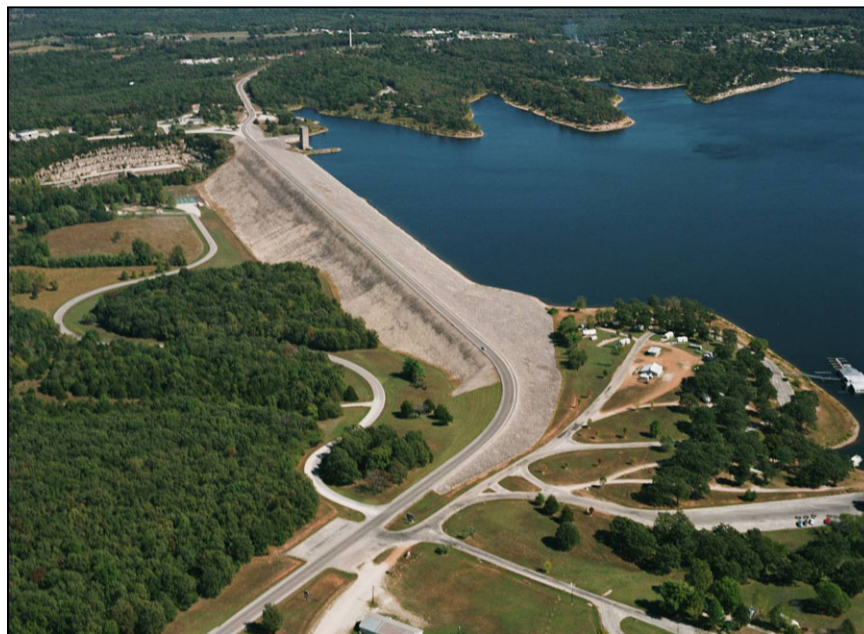
Figure A-76. —Aerial view of Pomme de Terre Dam.
