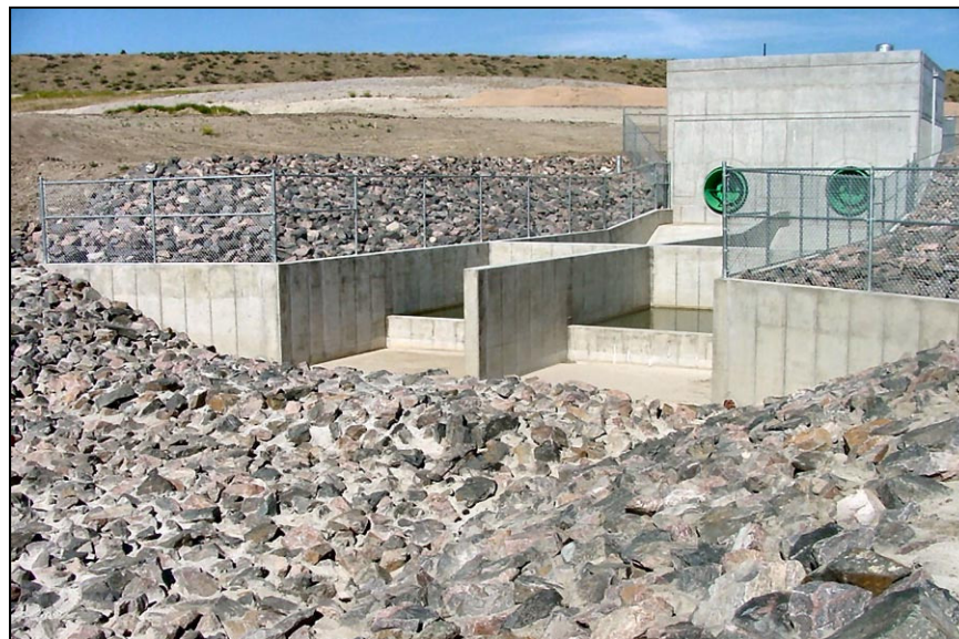
Figure 60. —Concrete-lined plunge basin with baffle wall, grouted riprap side slopes, and discharge channel. Flow discharges into the plunge basin from two 36-inch diameter fixed-cone valves.
