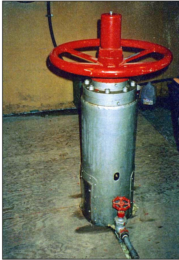
Figure A-3. —Handwheel control for sleeve valve. The handwheel requires 36\frac{3}{4} turns to fully open the valve from the closed position.
