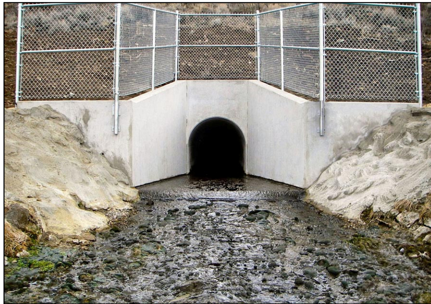
Figure 72.—A flared outlet transition.
