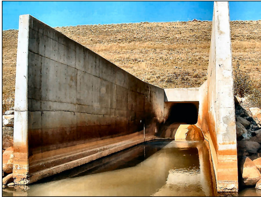
Figure 5. —Hydraulic jump stilling basin. Note the hydraulic jump flow pattern on the interior surface of the basin walls.
