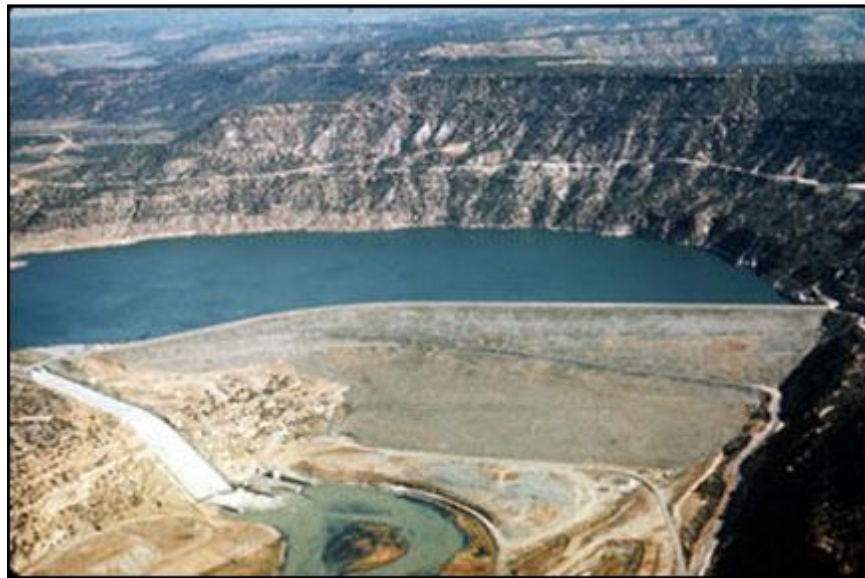
Figure A-53. —Aerial view of Navajo Dam. The hollow-jet-valve outlet works basin is located next to the spillway stilling basin.
