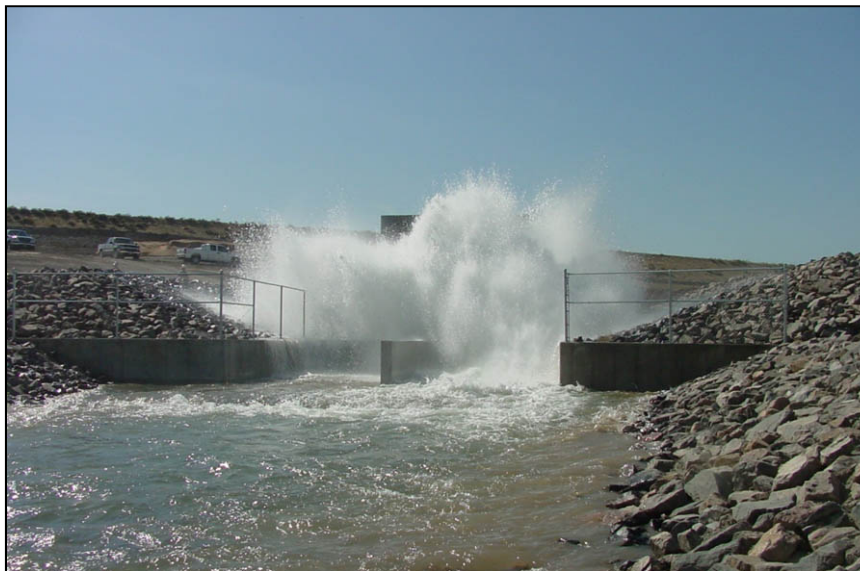
Figure A-102. —View looking upstream at the stream release facility with both fixed-cone valves operating each at 20 percent opening (total of 167 ft 3 /s).
