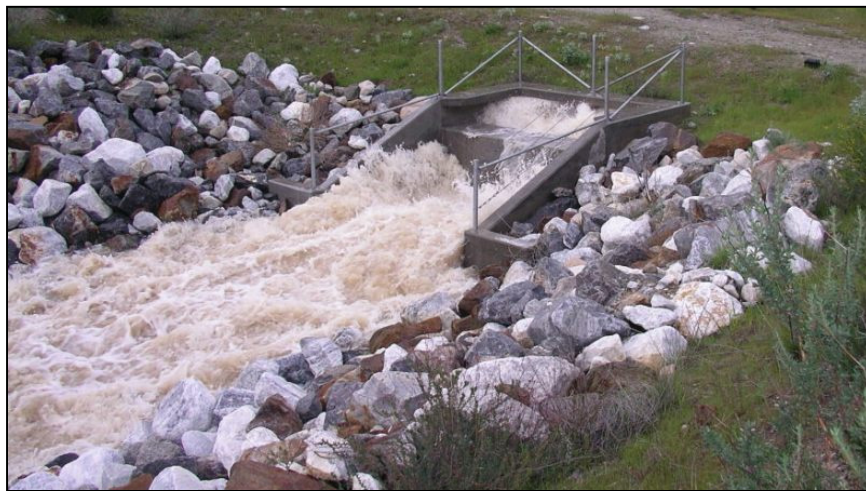
Figure A-93.—Same energy dissipator with flow ( 120 \text{ ft}^3/\text{s} ).
