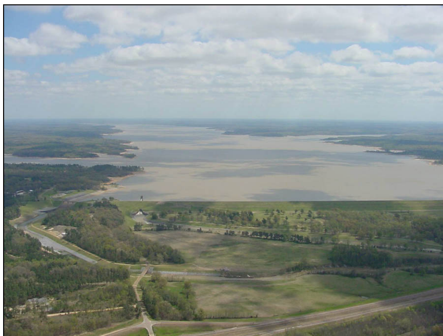
Figure A-15. —Aerial view of the downstream face of Enid Dam.
