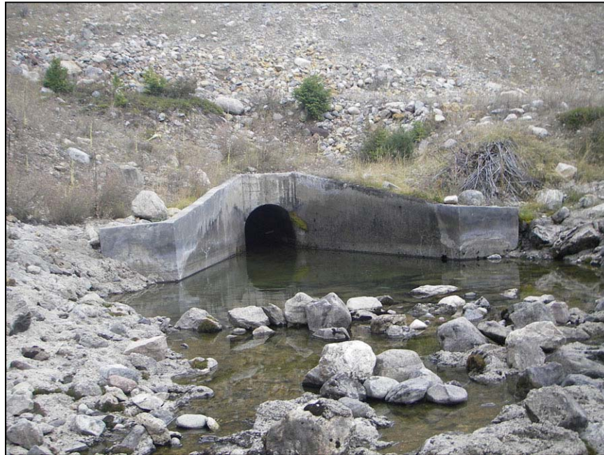
Figure 126. —The grouted riprap has performed well although some of the larger rocks in the foreground are displaced immediately downstream of the concrete apron.
