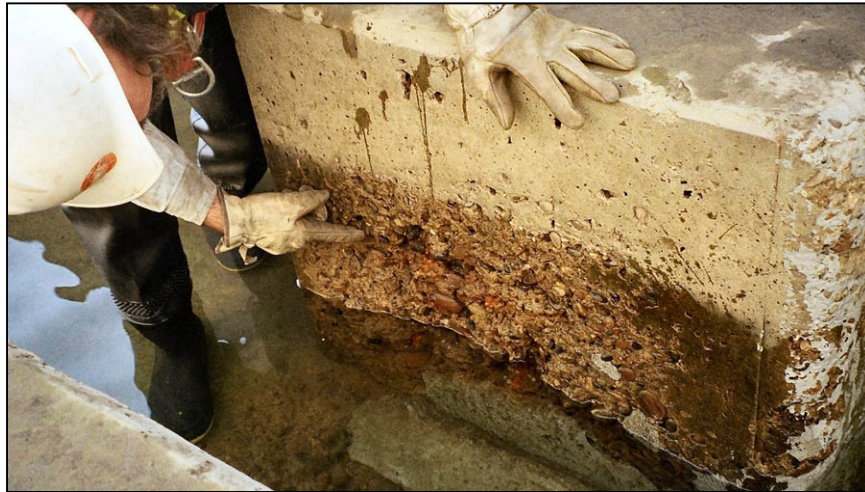
Figure 147. —Abrasion erosion damage at a dentate block.
