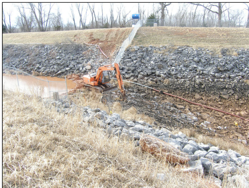
Figure A-60. —The contractor created a small earthen dike in the downstream river channel to facilitate unwatering of the stilling basin.
