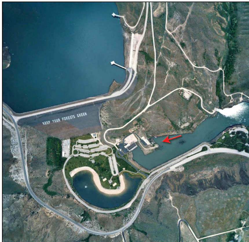
Figure A-43. —Aerial view of Lucky Peak Dam. The arrow denotes the location of the six slide gates and flip buckets.
