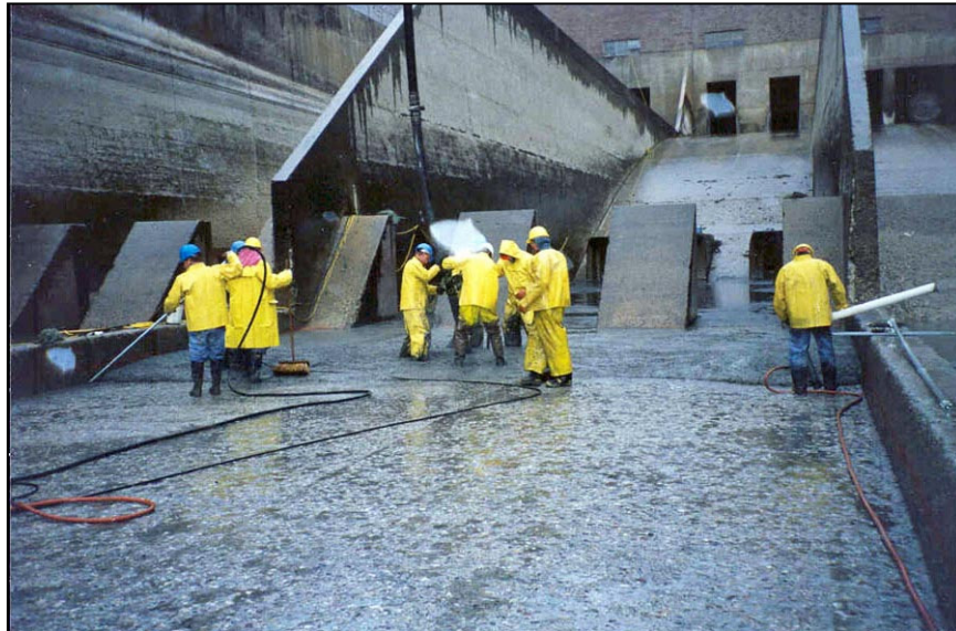
Figure A-73. —Closer view of concrete being placed.
