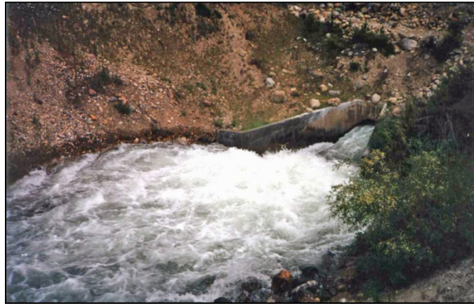
(a) The discharge is 270 \text{ ft}^3/\text{s} with an approximate Froude number equal to 1.6.
