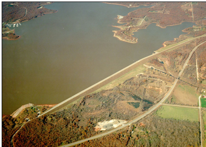
Figure A-59. —Aerial view of Norman Dam.
