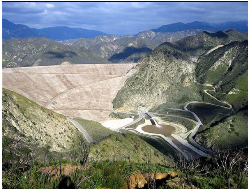
Figure A-84. —Seven Oaks Dam.
