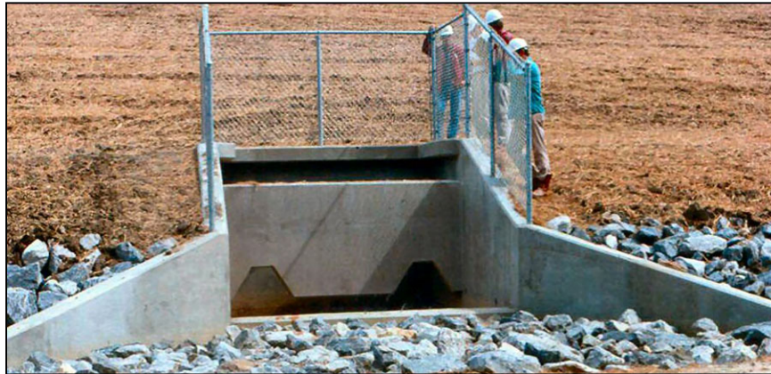
Figure 6.—A stationary baffle in an impact basin.
