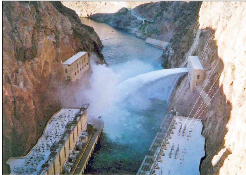
Figure 100. —68- and 90-inch diameter jet-flow gates discharging. Photo courtesy of URS Corporation.
