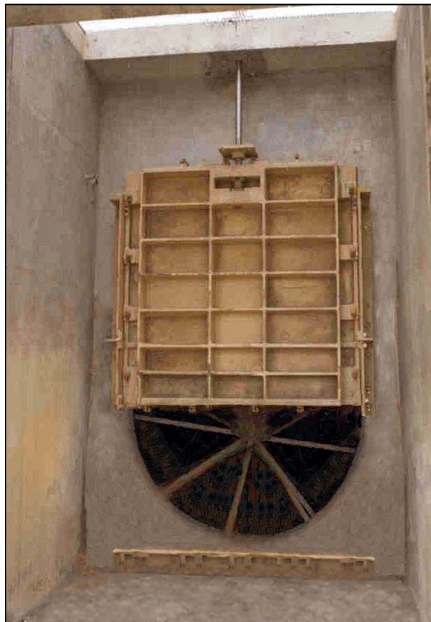
Figure 104.—Unbonneted slide gate.
