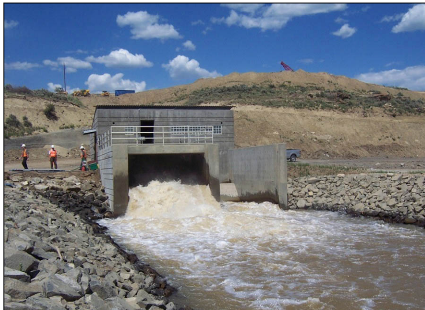
Figure A-22. —View of 42-inch diameter fixed-cone valve discharging at about 20 ft 3 /s.
