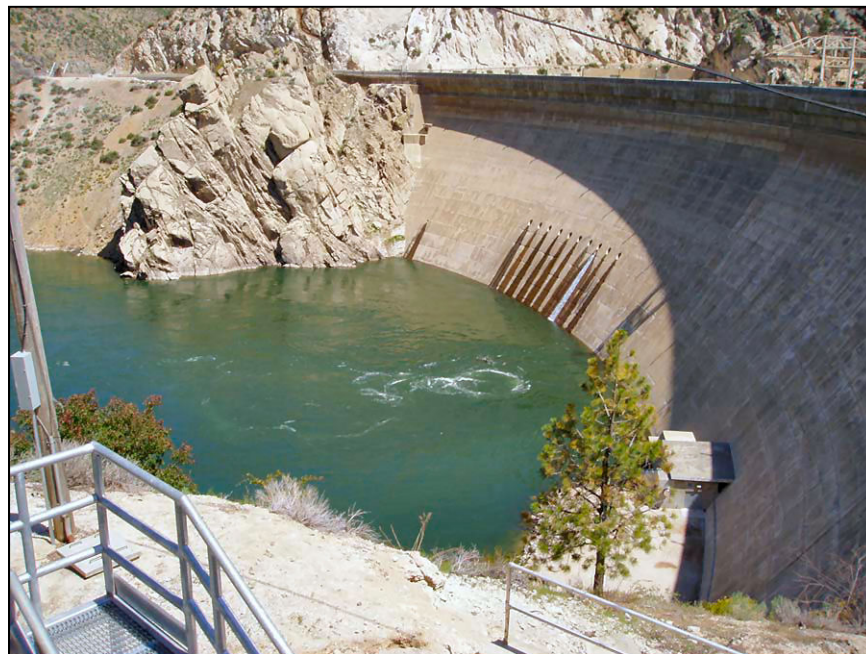
Figure 111.—Clamshell gates operating under 50 feet of submergence. No air was entrained during submerged discharge.
