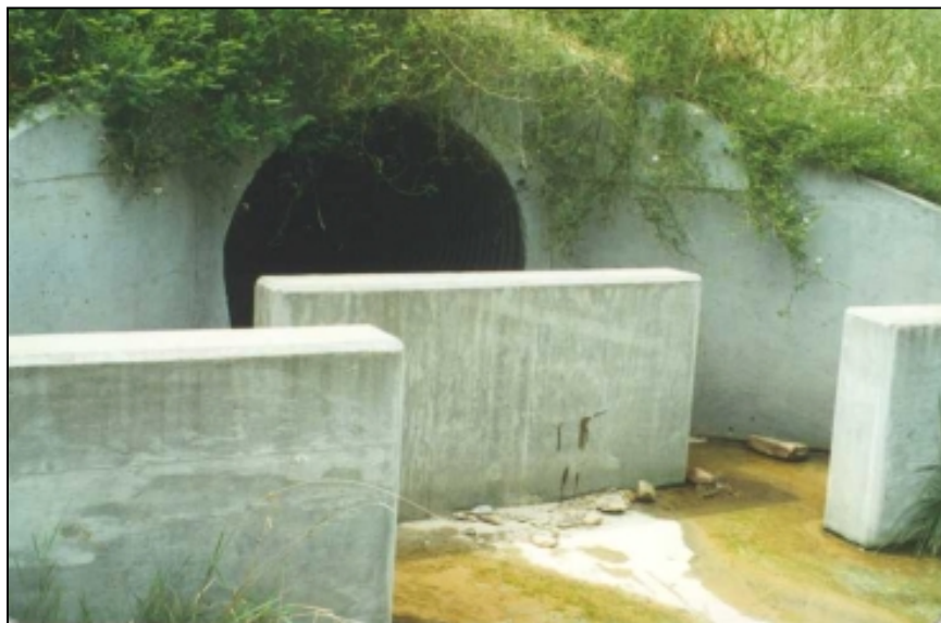
Figure 56. —A standard baffle basin.
