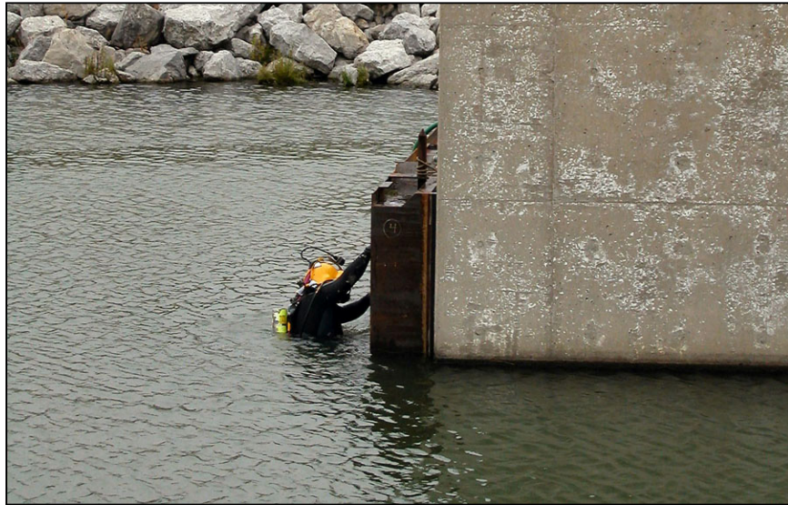
Figure 165. —Divers assisting with the installation of stoplogs at the downstream end of a stilling basin. Turnbuckles were attached to the stoplogs and basin. These held the stoplogs against the end of the basin walls until the basin was unwatered and the outside water pressure kept them in place. Rubber seals on the stoplogs prevented leakage.
