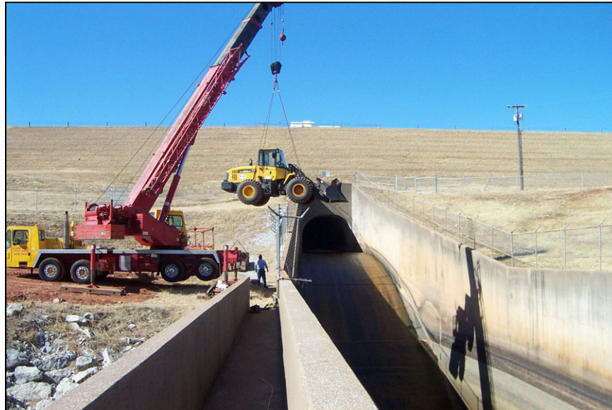
Figure A-62. —A crane was used to lower a front-end loader into the basin. The front-end loader was used to load debris into a metal container for removal.
