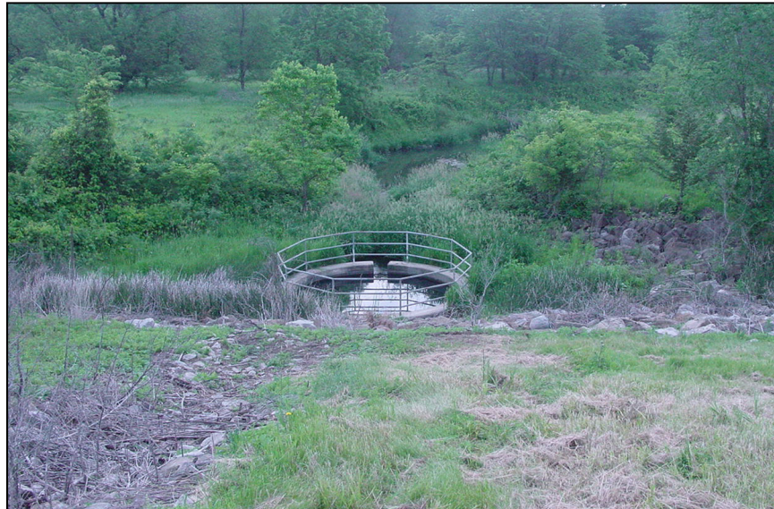
Figure 65.—Stilling well a at conduit outlet.
