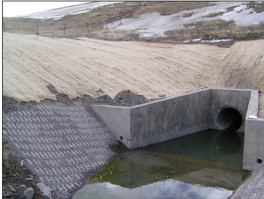
Figure A-58.—Replacement structure.
