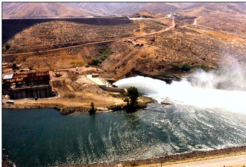
Figure A-44.—Discharge emerging from flip bucket operations.
