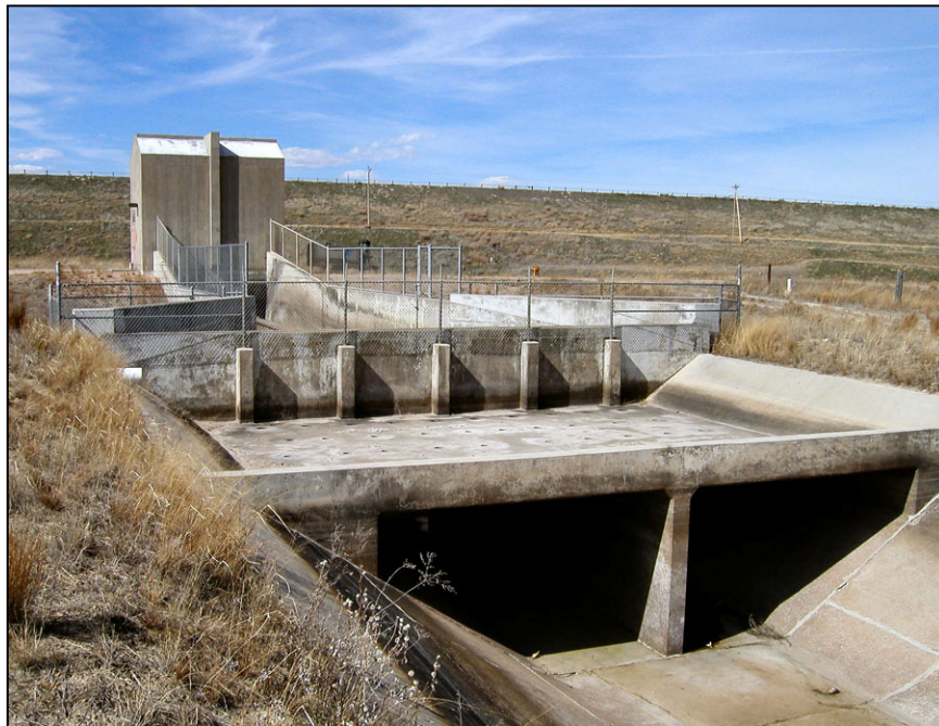
Figure 34. —This wave suppressor (also known as an underpass-type) was constructed after completion of the stilling basin to prevent unanticipated waves exiting the basin from overtopping the downstream canal lining. Overtopping could result in either undermining of the soil supporting the canal lining or introduction of uplift pressures beneath the canal lining. Note the formed openings through the deck of the wave suppressor.
