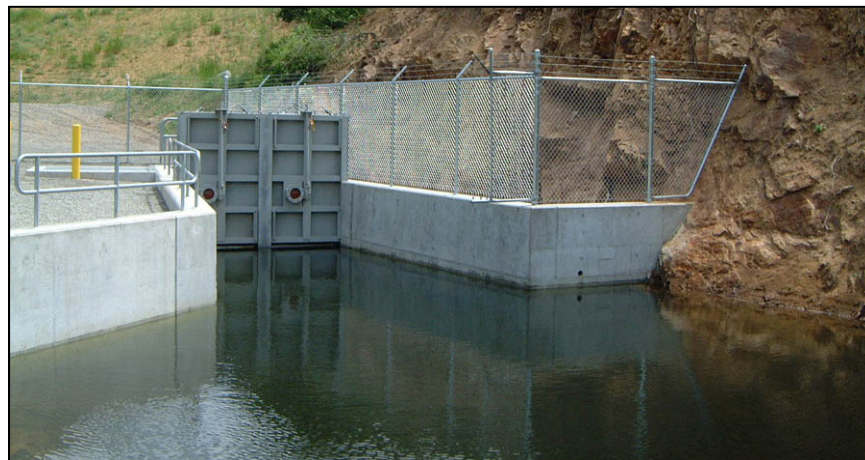
Figure 176. —Fencing at a stilling basin. The steep cliffs also provide an access deterrent.
