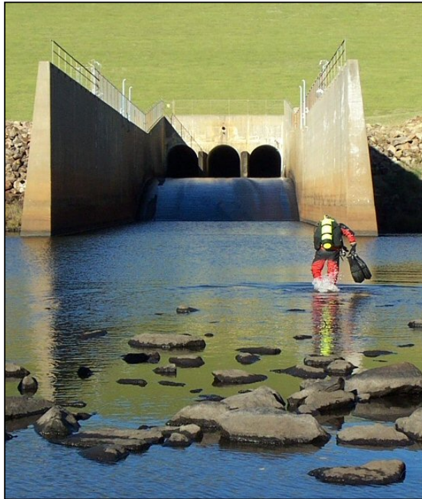
Figure 155. —A diver preparing to perform a stilling basin inspection.
