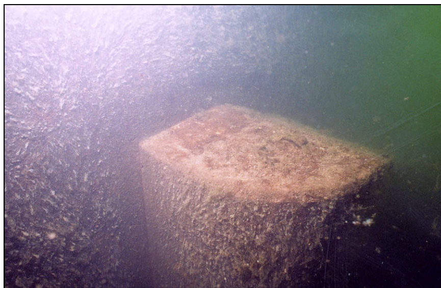
Figure A-13. —View looking downstream at far left dentate showing the general condition of outlet works stilling basin dentates. All dentates were in good condition with well defined edges and corners. No chipping of edges was noted.
