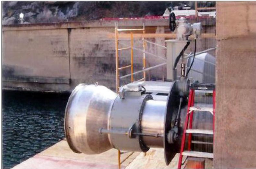
Figure 80. —Hooded fixed-cone valve. Photo courtesy of URS Corporation and Denver Water Board.
