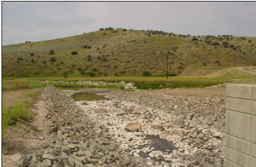
Figure A-24. —View of outlet channel from energy dissipation structure.
