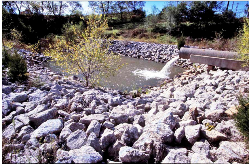
Figure 59. —A riprap-lined plunge basin.
