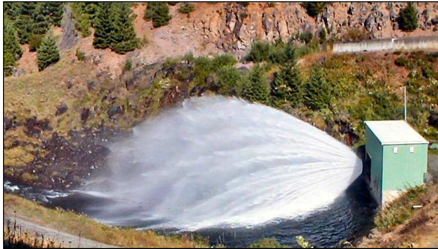
Figure 11.—Flow emerging from a Howell-Bunger valve.
