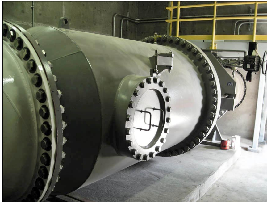
Figure 88. —The 48-inch diameter sleeve valve is located within a valve house and discharges directly into a horizontal stilling well. Photo courtesy of URS Corporation.
