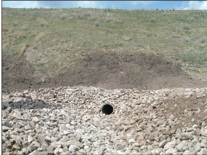
Figure 122.—A riprap apron used for erosion protection.
