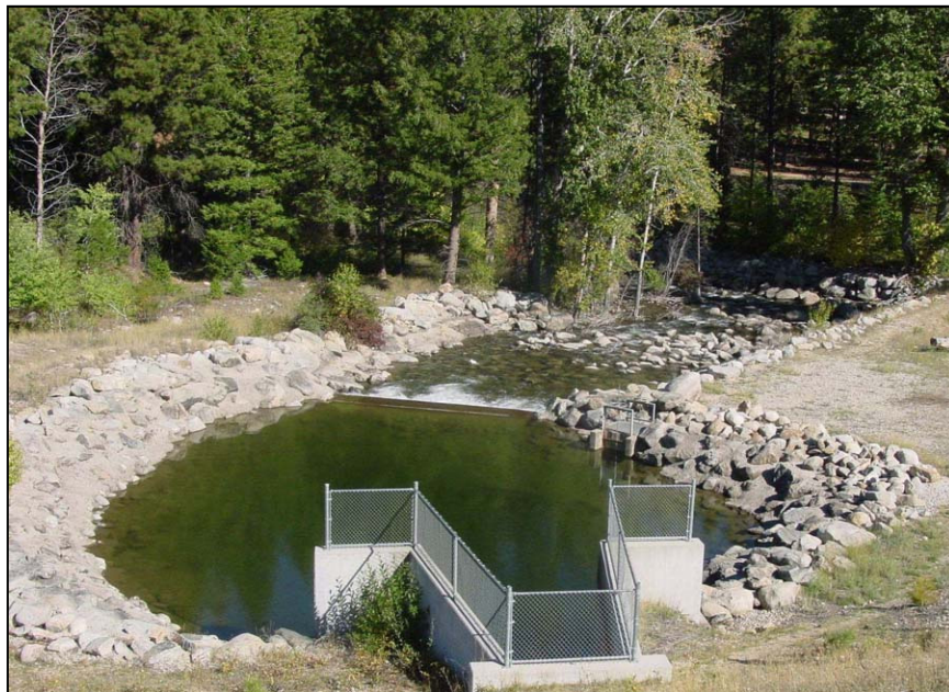
Figure 10. —Conduit outlet expansion.
