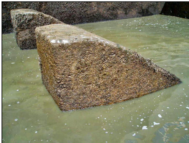
Figure 22. —Baffle blocks in a hydraulic jump stilling basin (flow is from left to right).
