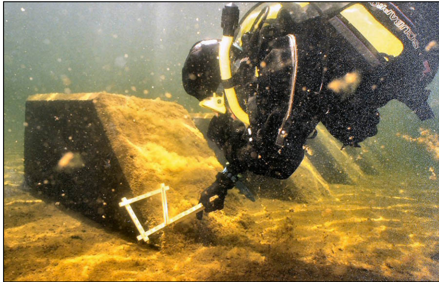
Figure 156. —A diver inspecting a baffle block.
