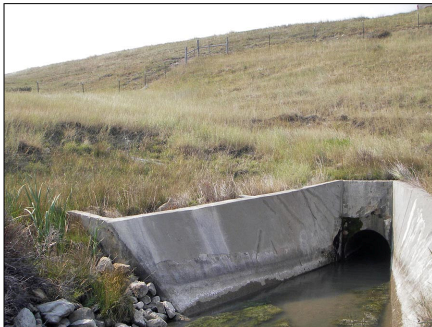
Figure A-56. —Original trapezoidal energy dissipator.
