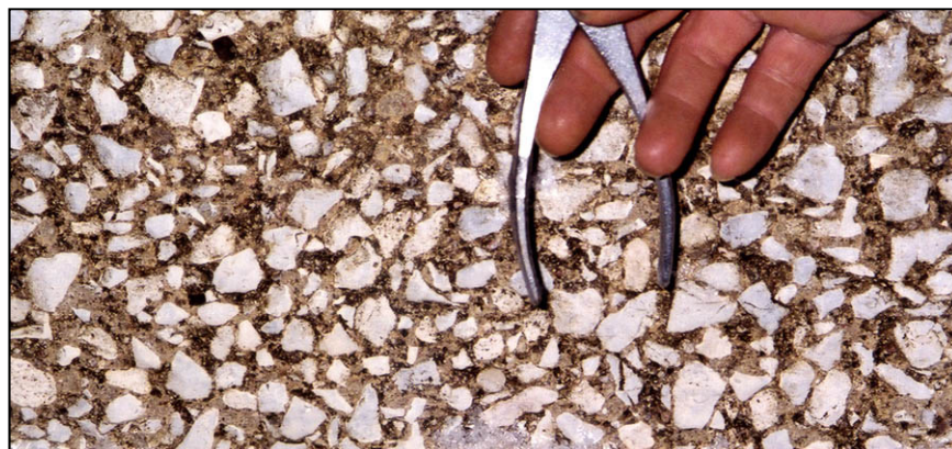
Figure A-123. —The exposed aggregate has been polished smooth by erosion.
