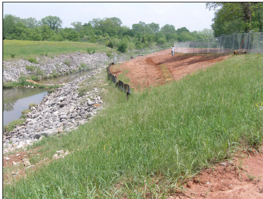
Figure A-65. —Slump area after cutting back slope. Sod is being placed to prevent erosion.
