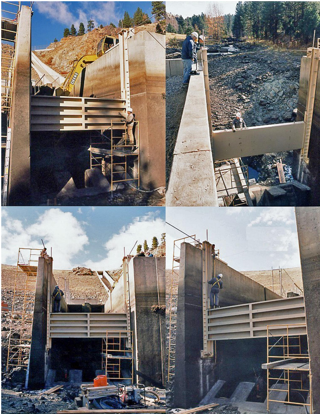
Figure A-51.—Prototype flow deflector installation at Mason Dam in October 2002.
