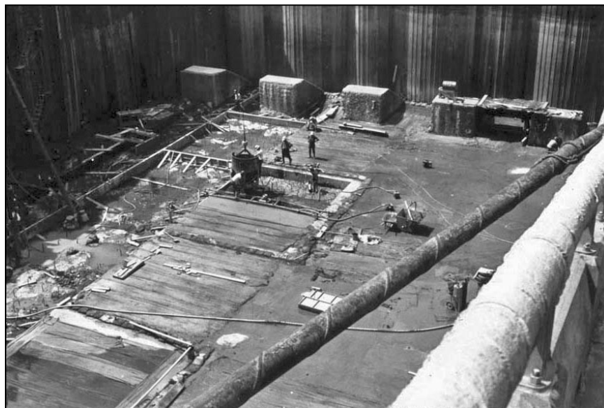
Figure A-40. —General view of repair operations.
