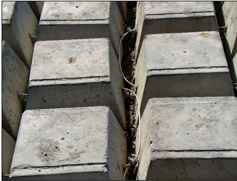
Figure 14. —Cable-tied concrete blocks.
