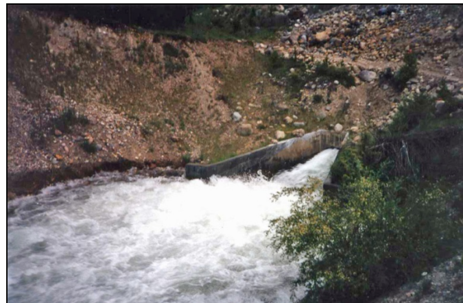
(b) The discharge is 400 \text{ ft}^3/\text{s} with an approximate Froude number equal to 2.0.
