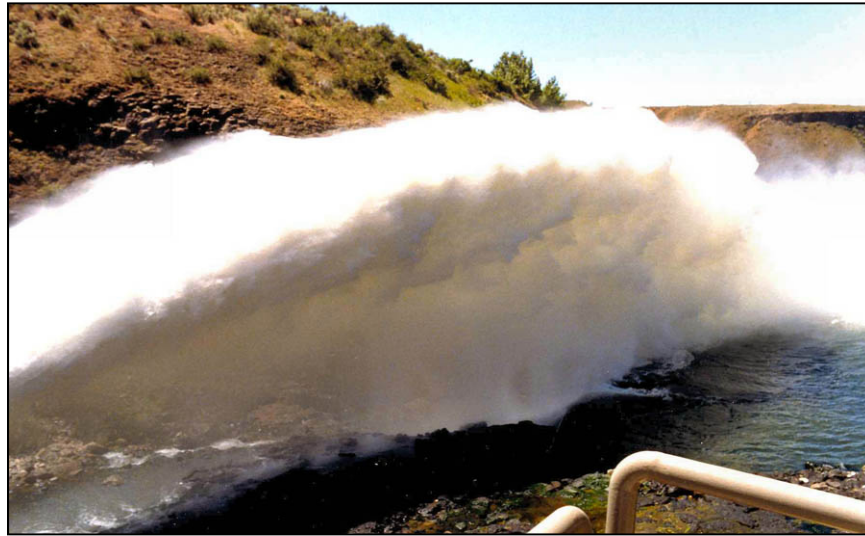
Figure A-45. —High velocity flow being directed downstream into the plunge basin.
