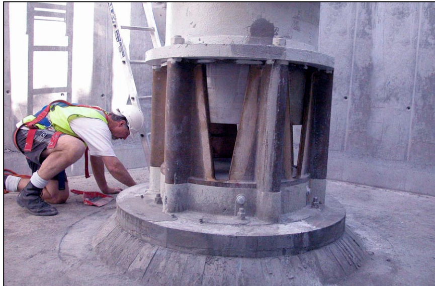
Figure 91. —Bottom discharge of a submerged discharge valve. Note the V port openings.
