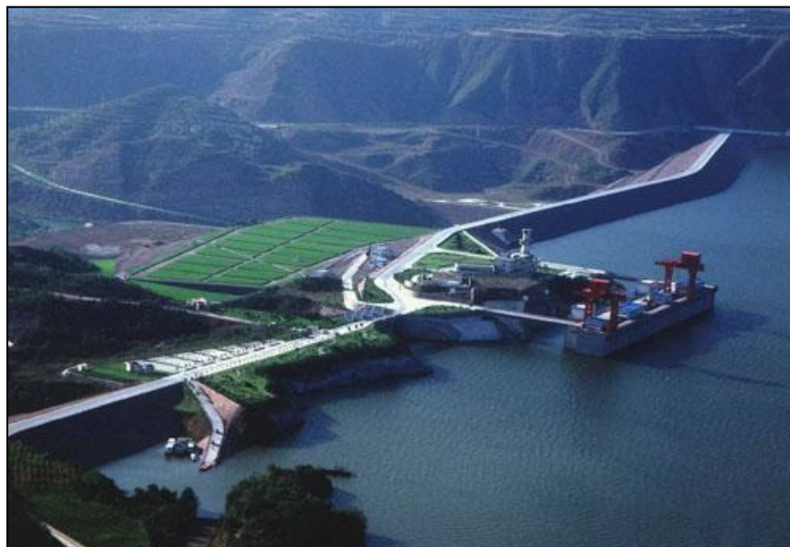
Figure A-130.—Aerial view of Xiaolangdi Dam.
