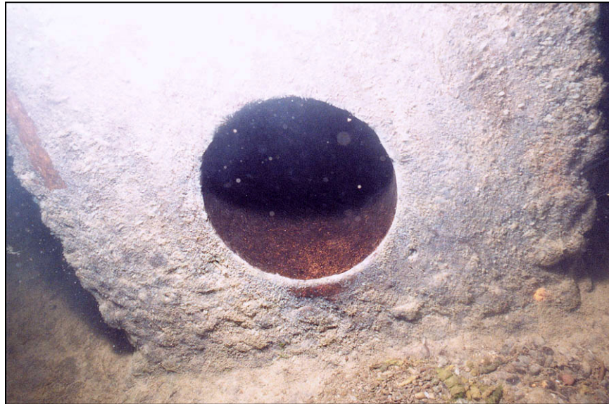
Figure A-11. —View looking upstream at outlet works stilling basin left chute block underdrain. The drain is clear and flowing. Note edge relief of the chute block and the exposed vertical rebar on the left side of block. Concrete erosion of block is approximately 1.5 to 2 inches.
