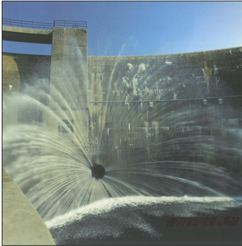
Figure 74.—Fixed-cone valve discharging at a small opening.
