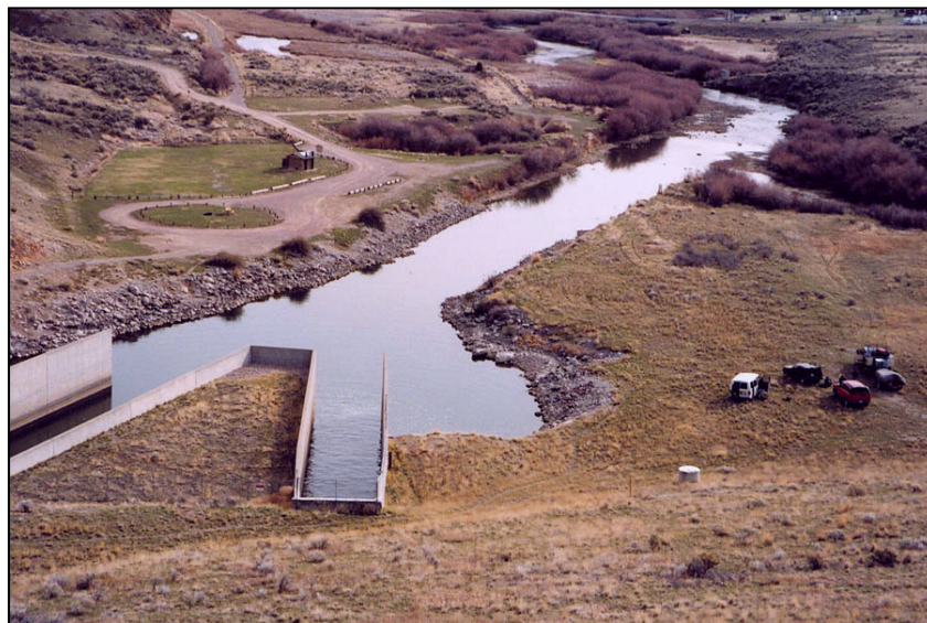
Figure A-9. —View looking downstream from top of dam with outlet works stilling basin in middle and spillway stilling basin to the left.
