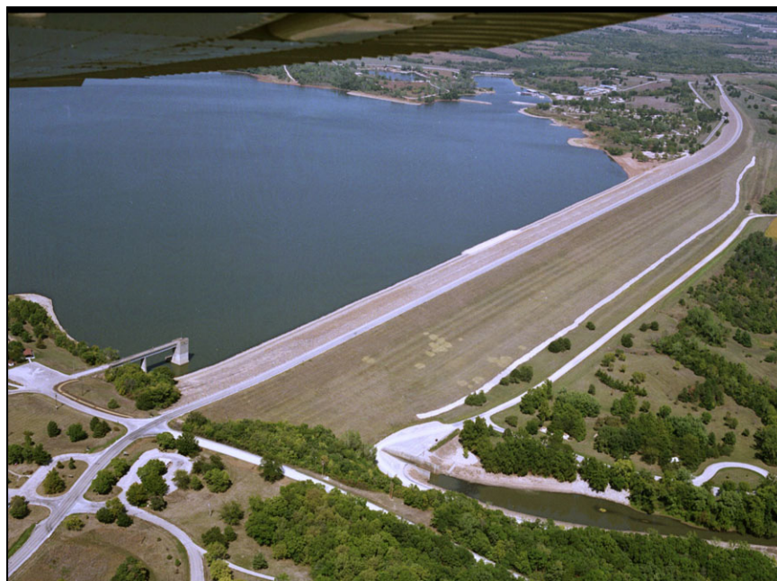
Figure A-80.—Aerial view of the downstream face of Pomona Dam.
