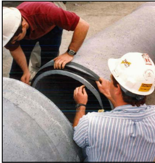
Figure 79. —A rubber gasket is installed at the spigot end of the precast concrete pipe.
