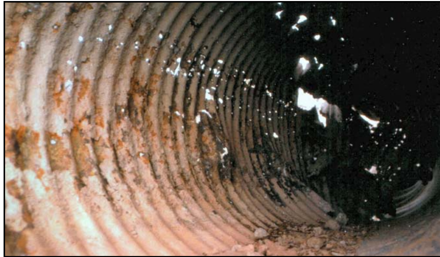
Figure 159. —The holes in this CMP conduit were clearly visible after removal. The conduit was considered to be so severely corroded that sliplining was not an option and it was removed and replaced. Photo courtesy of Maryland Dam Safety Division.
