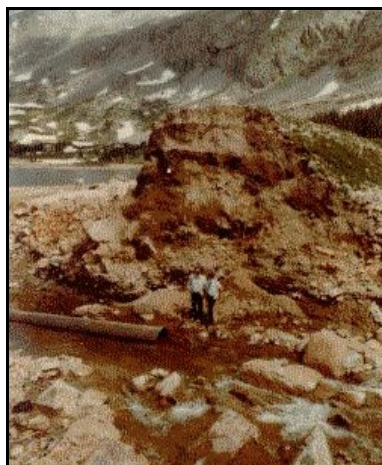
Figure B-48. —Left side of the breached Lawn Lake Dam.
