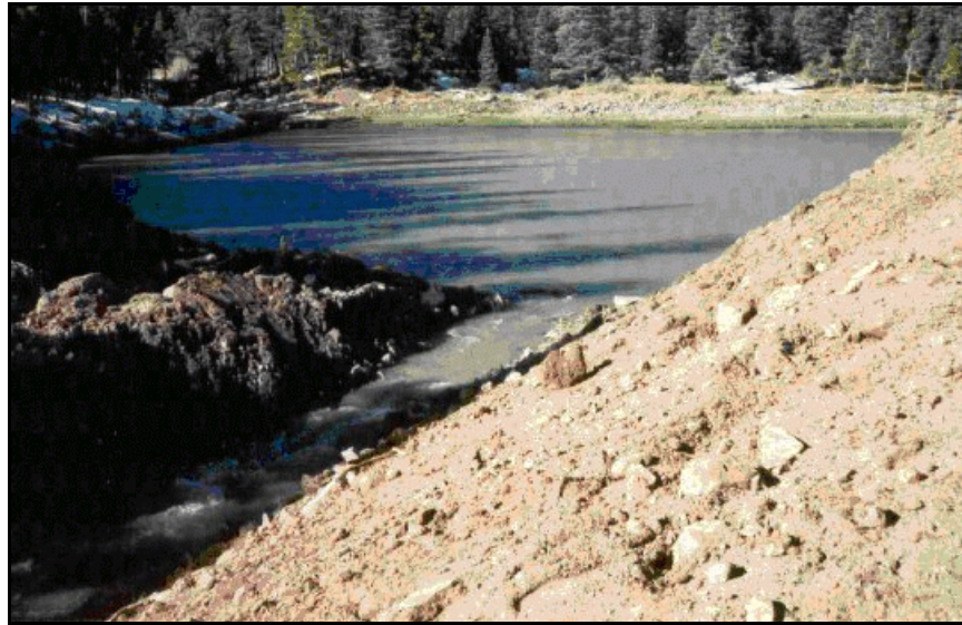
Figure B-18. —Initialization of the breach in the embankment dam near the left abutment.
