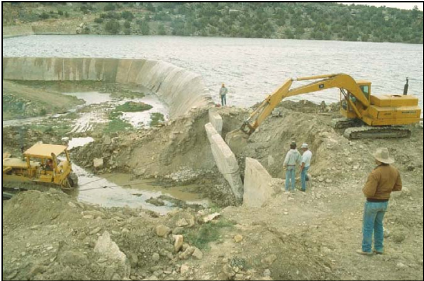
Figure 155.—Spillway being partially breached to lower the reservoir.
