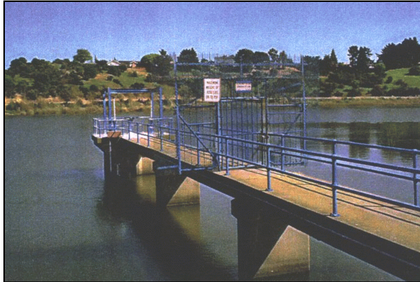
Figure 38. —A footbridge or access bridge is often required to operate gates or valves located at the intake tower.
