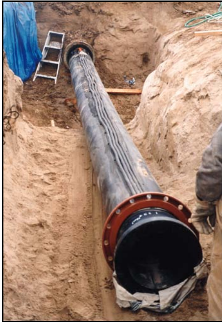
Figure B-75. —HDPE slipliner being installed at Turtle (Twin) Lake Dam. Note the HDPE grout lines welded onto top of new liner. The end flange was used to attach the two different sized liners together.
