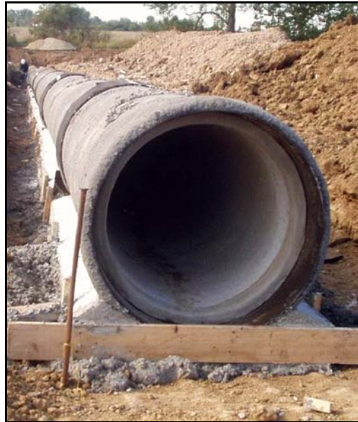
Figure 60. —Precast concrete using bedding as support.
