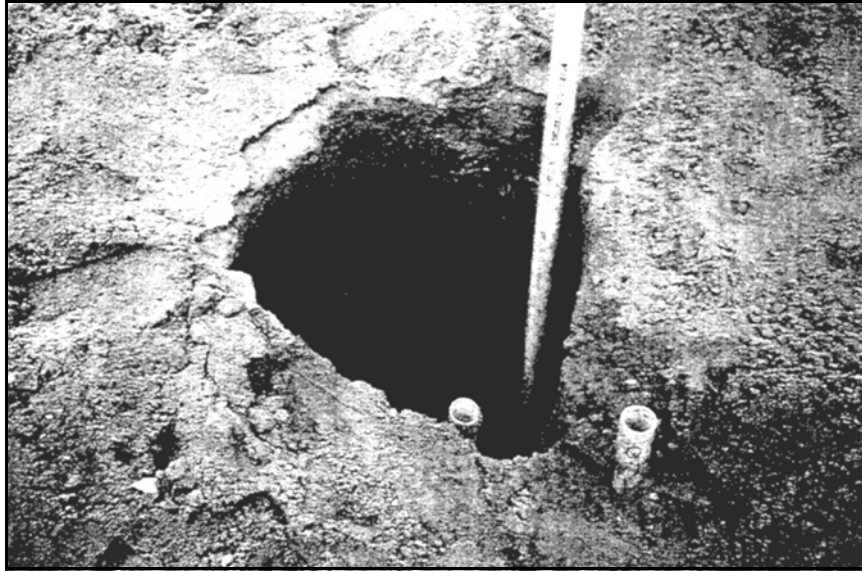
Figure 189. —A very large surface void appeared directly above a test microtunneling installation when the operator stopped advancement of the machine and briefly allowed the slurry pump to continue to circulate the drilling mud. The void appeared in backfill surrounding some test instruments, some of which appeared to support the adjacent soils.
