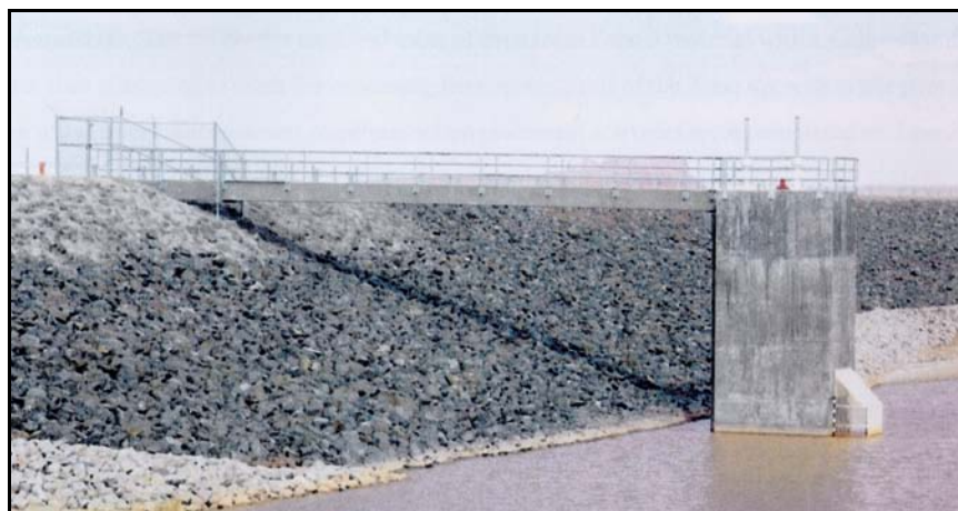
Figure 42. —Typical outlet works intake structure.
