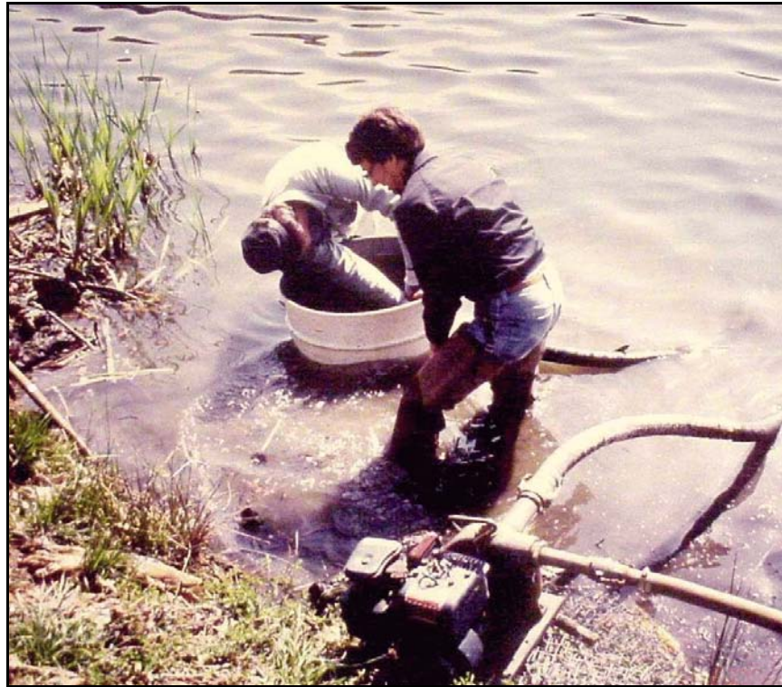
Figure 153. —The upper portion of a small metal pipe riser structure was removed with an acetylene torch. The riser was isolated from the pool by surrounding it with a large drum pressed into the soil. A pump was used to remove the water between the drum and the riser so that the work was completed in the dry.
