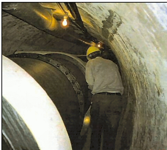
Figure 37. —A steel pipe is located within a larger downstream access conduit.
