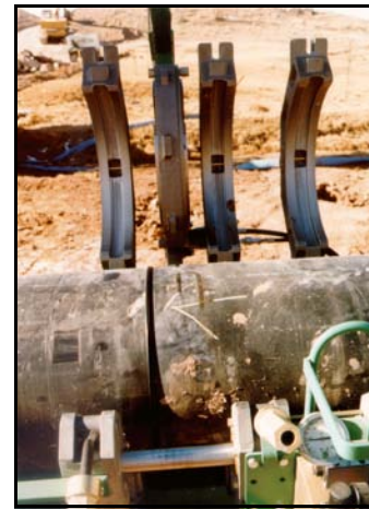
Figure 164. —Finished fusion welded joint.
