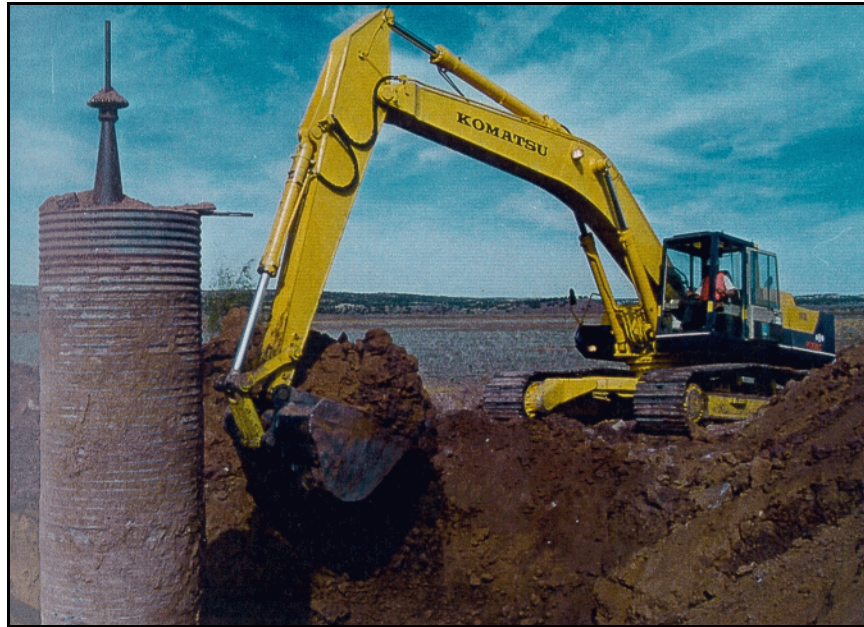
Figure 186. —Excavator removing the intake structure for an existing outlet works.
