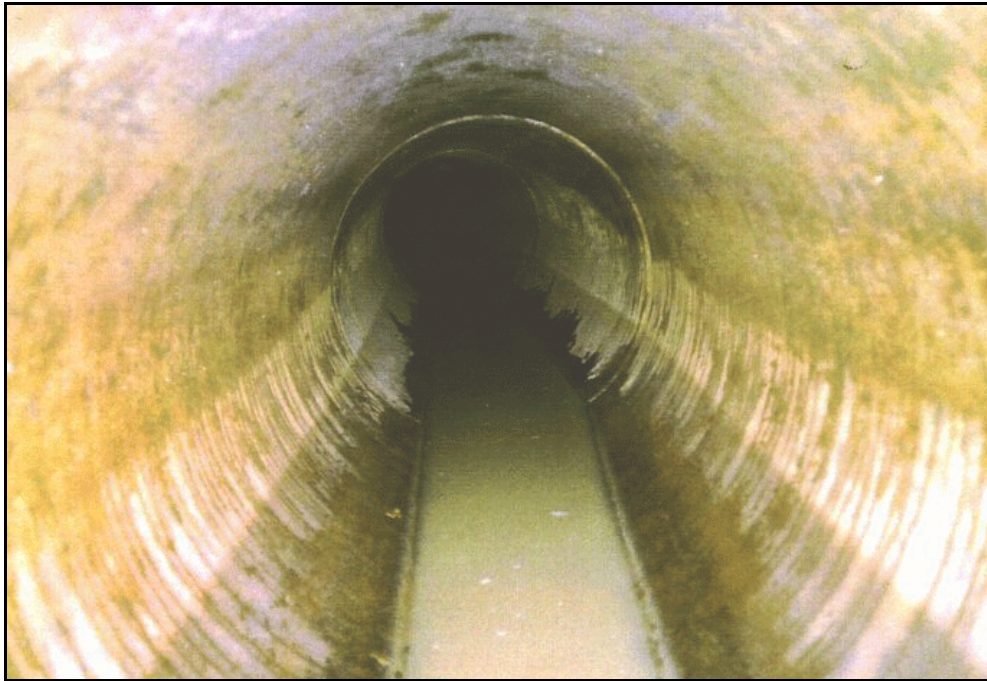
Figure 54. —An example of the interior of conduit shape A.
