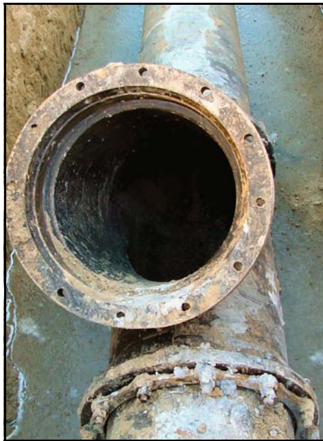
Figure 29. —Flanged joints of ductile iron pipe improve the watertightness of the joint.
