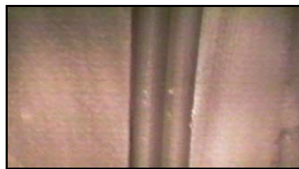
Figure 165. —Interior view of finished joint bead.
