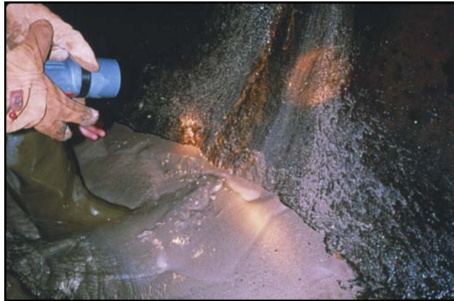
Figure 97. —Soil particles being carried into an outlet works conduit through a joint.
