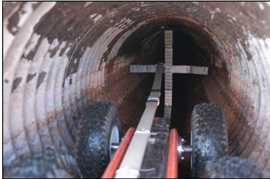
Figure 160. —Crossbar template attached to a CCTV camera-crawler to check for irregularities in the CMP conduit.
