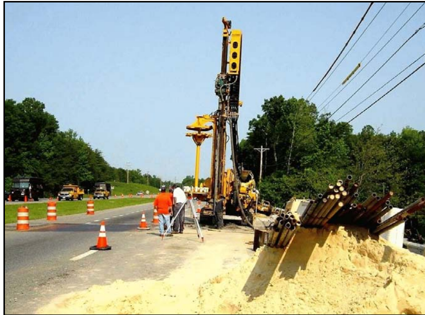
Figure B-32. —The failed CMP and voids were filled with a stiff compaction grout.
