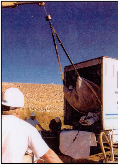
Figure 182. —Unloading the CIPP liner prior to installation.
