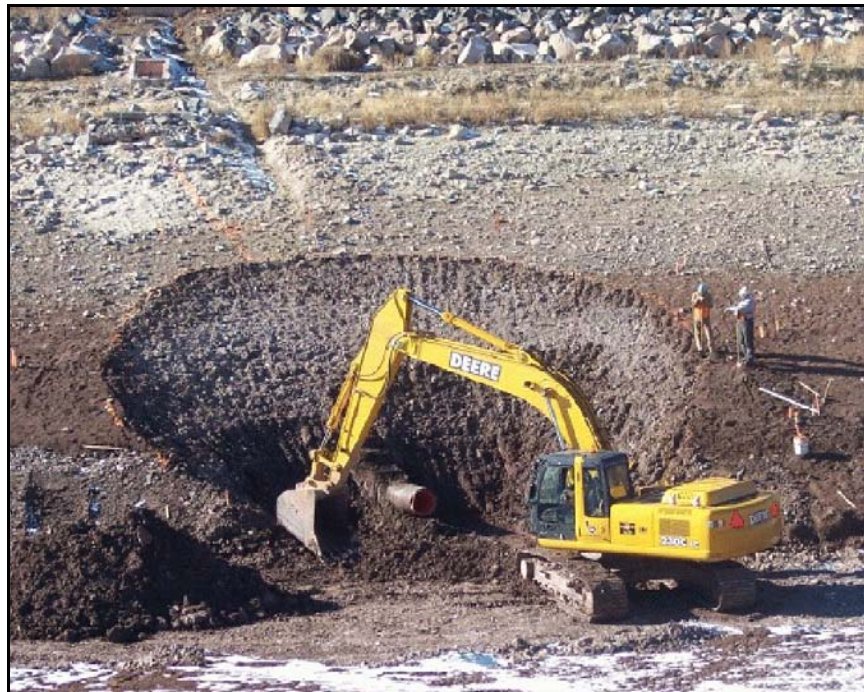
Figure 170. —The intake structure has been removed as part of a conduit renovation.
