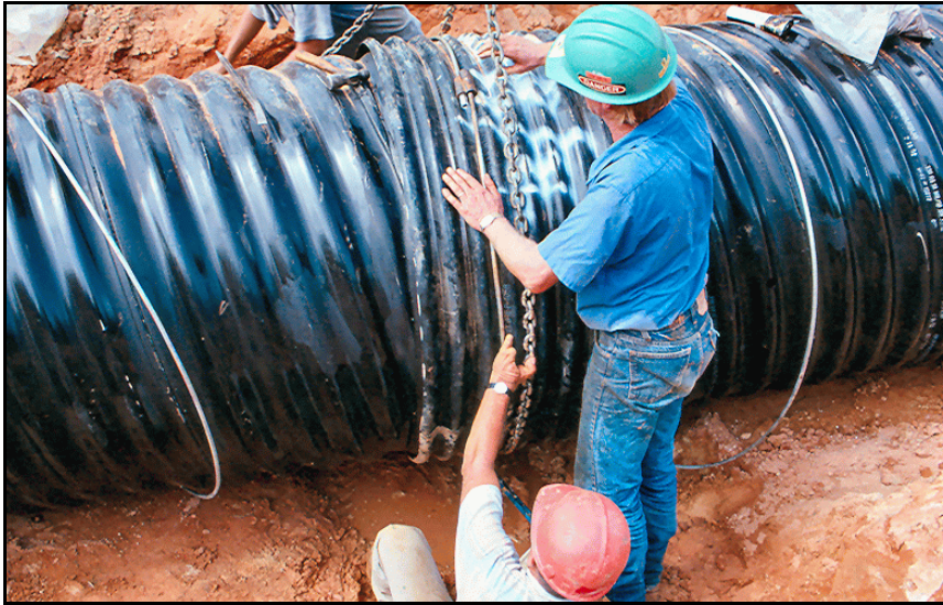
Figure 31. —A CMP conduit being installed.
