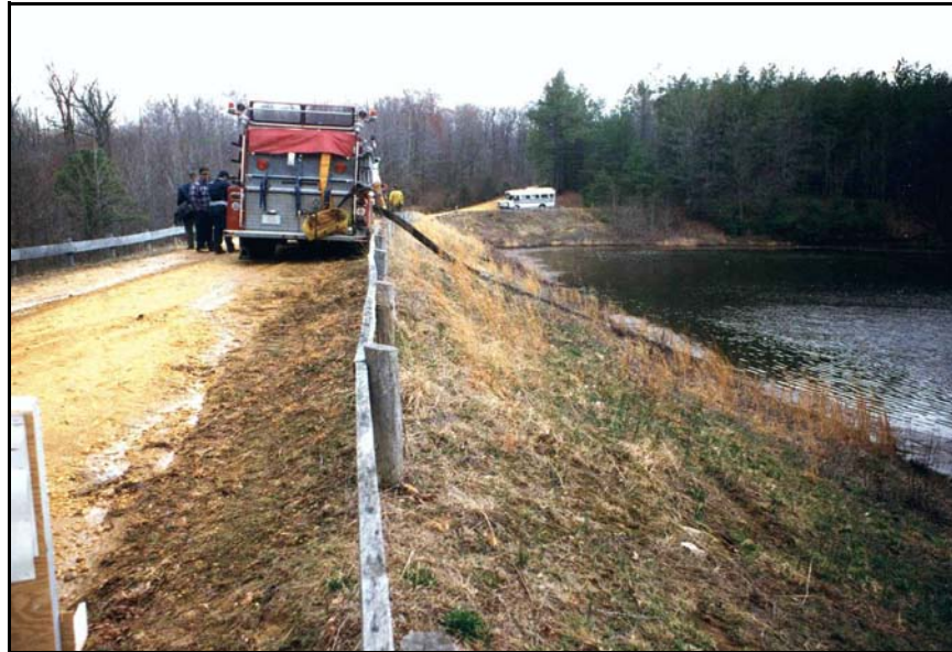
Figure 152. —All available resources may need to be utilized to drain the reservoir in an emergency. Here, the local fire department assists in draining a lake during a thunderstorm after the 45-year old CMP spillway collapsed.
