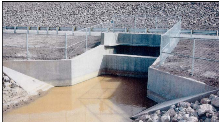
Figure 43. —Typical outlet works terminal structure.
