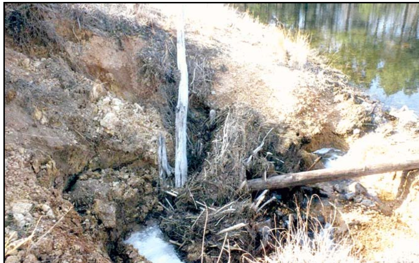
Figure 154. —Care must be taken to ensure that debris does not clog spillway after removal of the riser.
