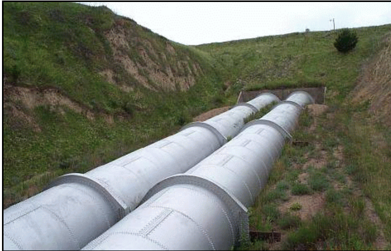
Figure 41. —Penstocks extending through an embankment dam.
