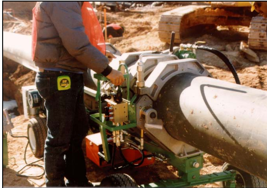
Figure 163. —HDPE pipe joint being fusion welded.
