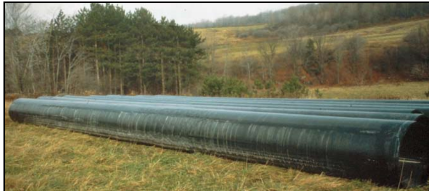
Figure 24. —HDPE pipe to be used for sliplining of an existing conduit.
