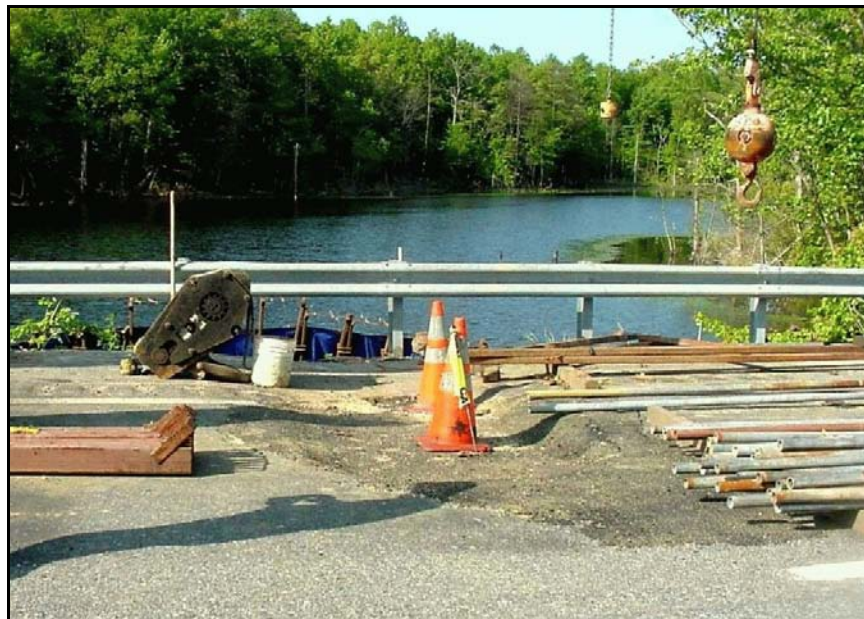
Figure B-29. —A sinkhole, which appeared in a heavily traveled roadway above a 20-year old CMP spillway, was filled with asphalt. Part of the roadway was closed when the asphalt patch subsided a few hours later.
