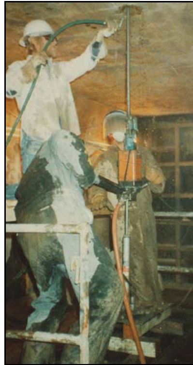
Figure B-45. —Grouting operations within the conduit.
