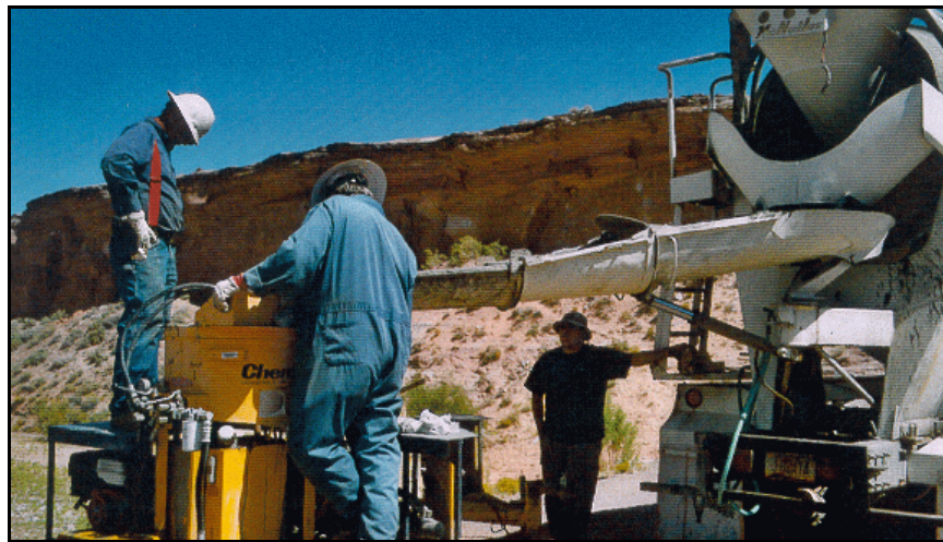
Figure B-62. —Grout mix being conveyed directly into the grout mixer from the transit mixer truck.
