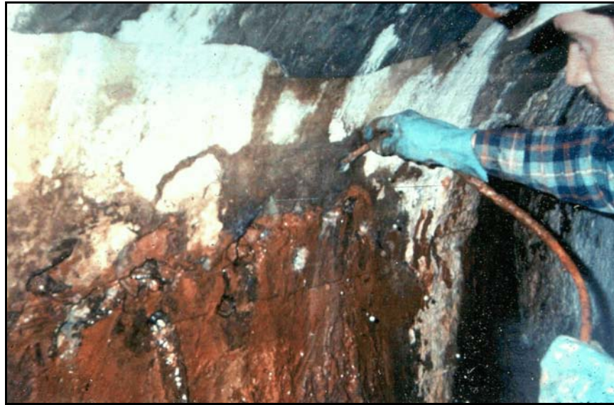
Figure 192. —Injection of urethane grout to stop leakage.
