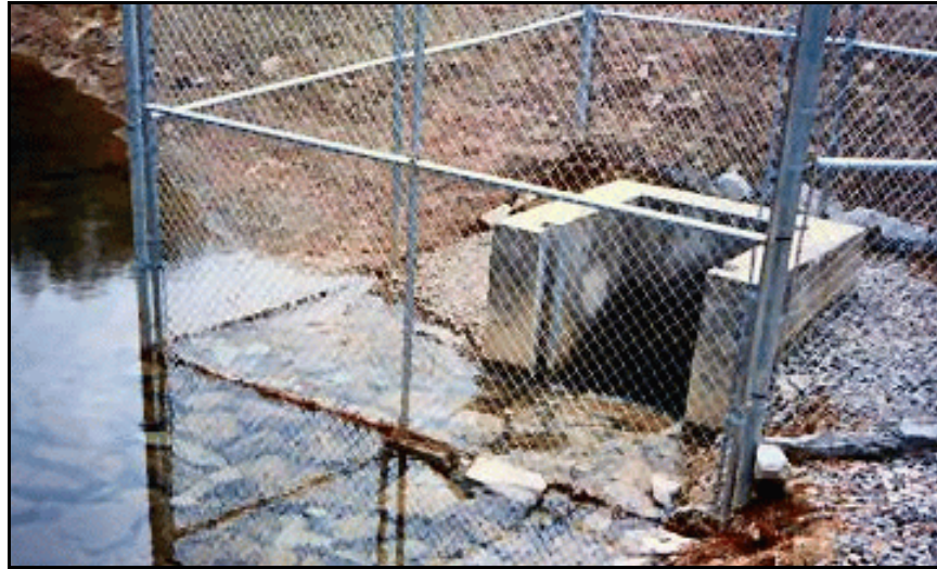
Figure 13. —An example of a decant intake structure.
