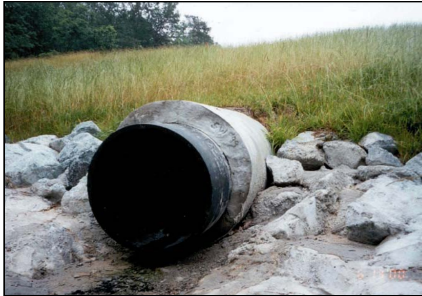
Figure 176. —Completed HDPE slipliner in existing CMP spillway conduit. Photo courtesy of Maryland Dam Safety Division.
