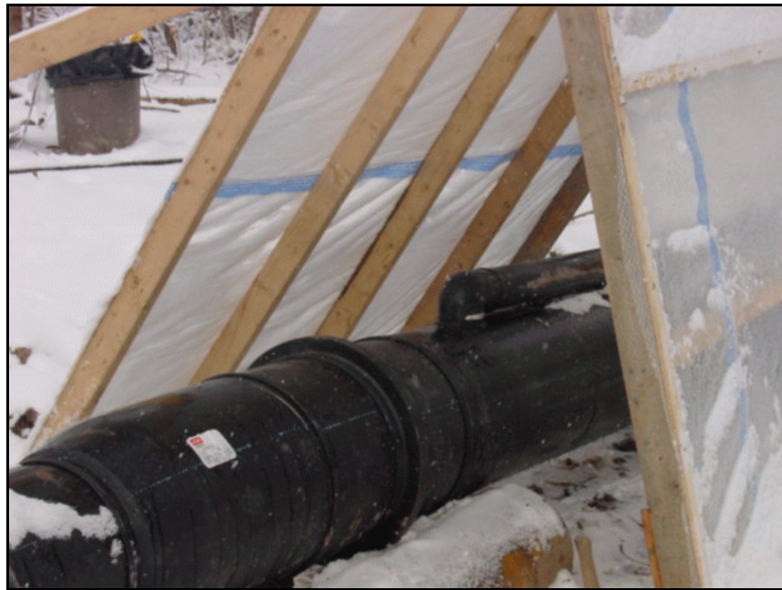
Figure 166. —Cold weather shelter constructed for joining sections of HDPE pipe.
