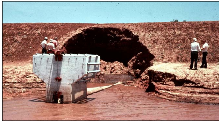
Figure 5. —Embankment dam failure caused by internal erosion of earthfill near the conduit. Flow was not directly along the contact between earthfill and conduit, but in the earthfill away from conduit. Hydraulic fracture in highly dispersive clay embankment soils caused the failure. The embankment design included antiseep collars, but not a filter diaphragm.
