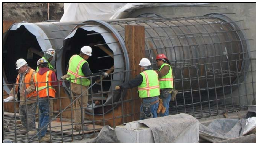
Figure 53. —A multibarrel outlet works conduit under construction.
