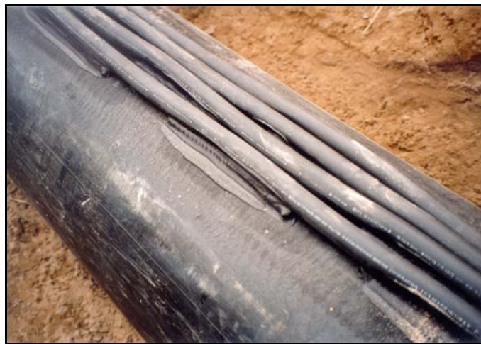
Figure 168.—HDPE grout pipe attached to HDPE slipliner.
