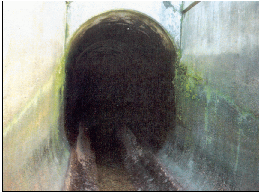
Figure 58. —An example of the interior of conduit shape E.
