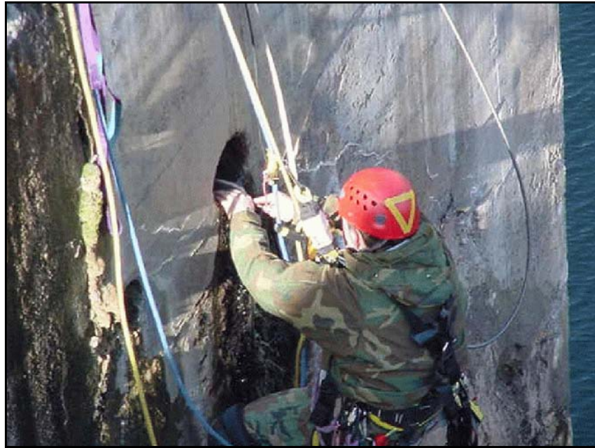
Figure 124. —Climber performing an inspection on a terminal structure wall.
