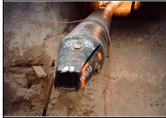
Figure B-76. —Upstream end of the HDPE slipliner modified to act as a pulling head.
