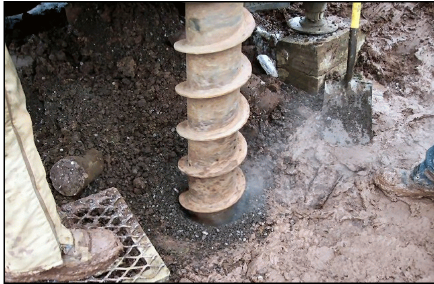
Figure 198. —An auger is being used to drill within an embankment dam.
