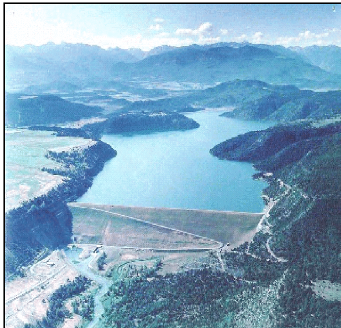
Figure B-65. —Aerial view of Ridgway Dam, Colorado.
