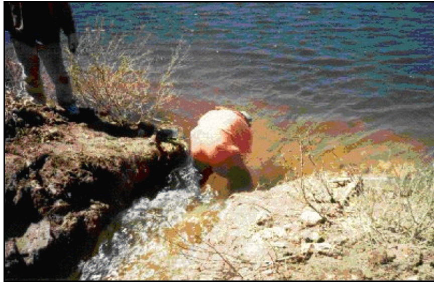
Figure B-40. —Deepening of the initial breach channel.
