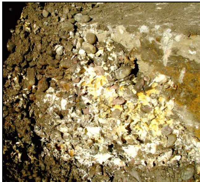
Figure 136. —Close coordination between the forensic team and contractor allowed for careful study of how polyurethane grout injected into the deteriorated joints of a conduit flows through surrounding backfill. In this case, the forensic investigation showed the injection of grout was relatively successful in sealing the joints of the conduit.
