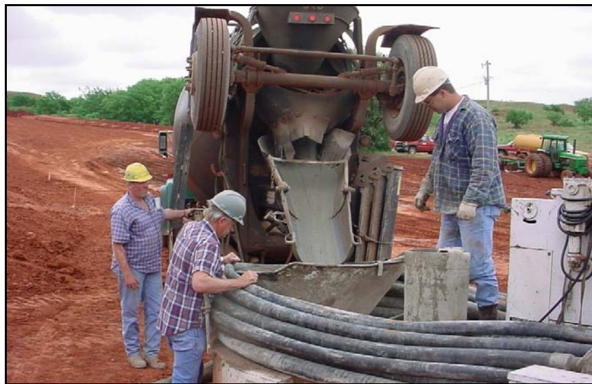
Figure 200. —Grout being delivered to the pumping truck.
