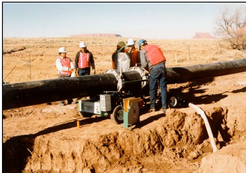
Figure B-68. —Heat fusion of an HDPE pipe joint.
