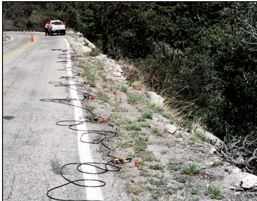
Figure 138. —Seismic tomography being used on an embankment dam. Photo courtesy of URS Corporation.
