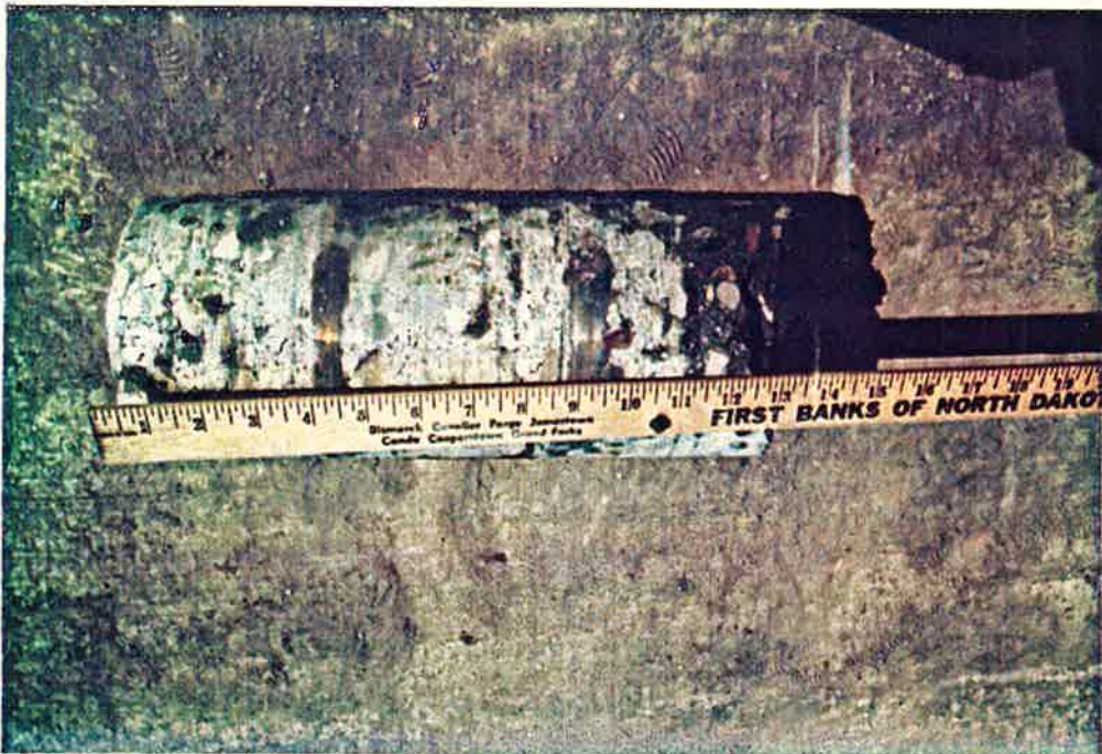
Photo No. 26 7-30-84 Close-Up View of 6-Inch Diameter Core Sample Removed From Structural Floor
