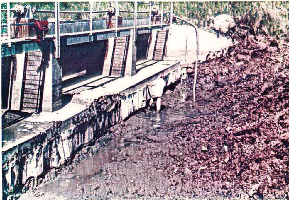
Photo No. 4 - Excavation and Pumping Operations Nearing Completion 6-27-84
