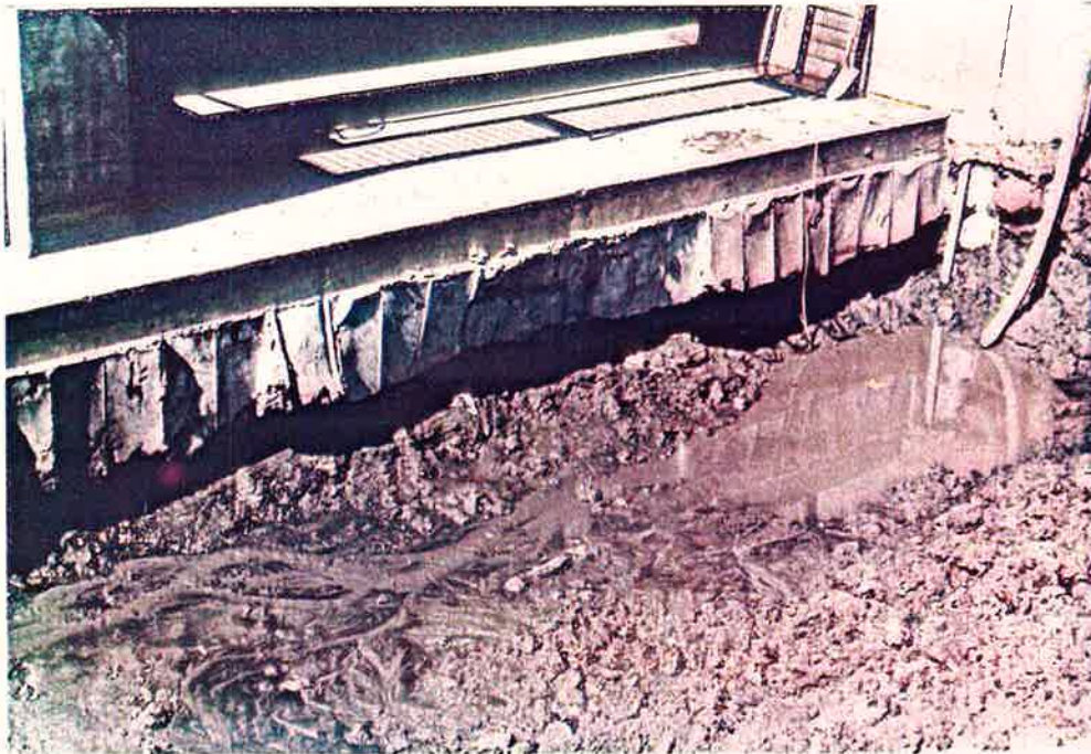
Photo No. 6 - Close-up View of Upstream Wall West Portion of Structure 6-27-84
