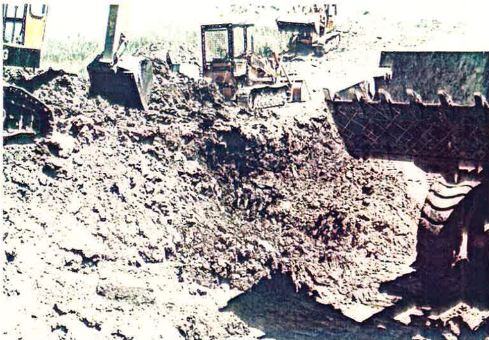
Photo No. 14 - Construction Equipment Upper Left: Warner Swasey Excavator Upper Middle: Case 350 Crawler Tractor Upper Right: JD555 Crawler Tractor Lower Right: JD644-B Loader 7-2-84
