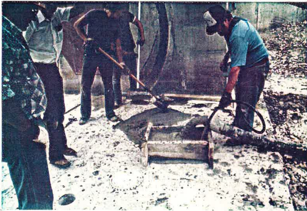
Photo No. 31 8-3-84 Another View of Concrete Simultaneously Being Pumped and Vibrated into the Structural Foundation. The Man Wearing the Blue Shirt is Don Dahl, Owner and Manager of Dahl's Industrial Tool Company, West Fargo, North Dakota
