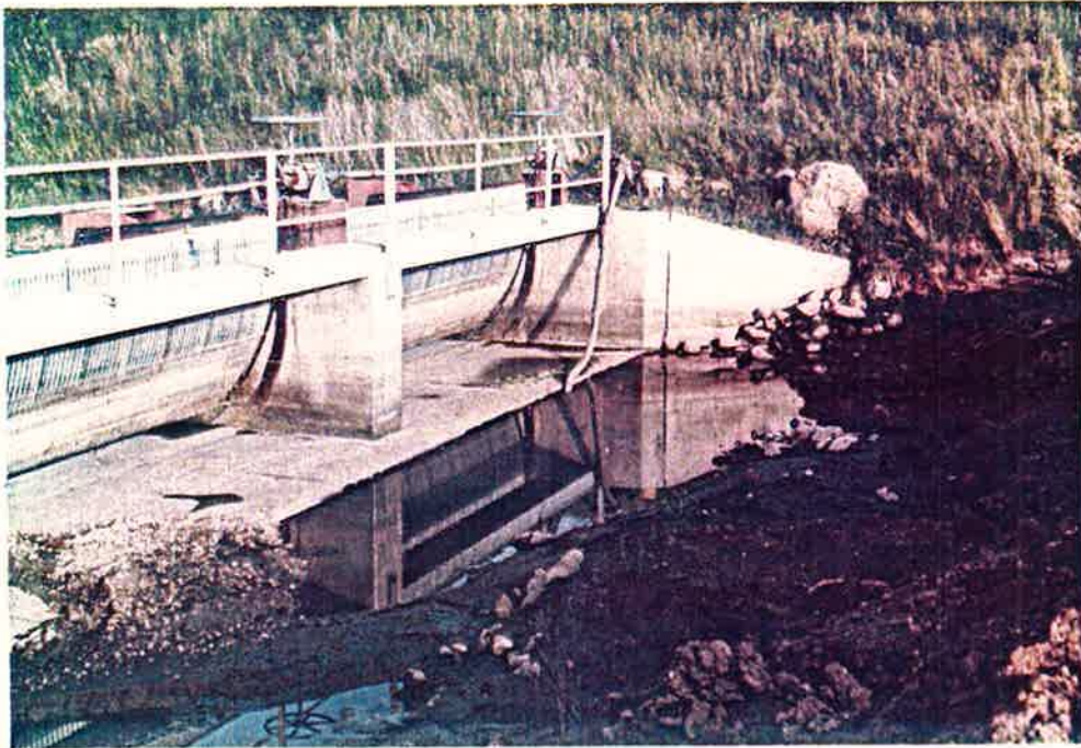
Photo No. 2 - Pumping Operations Begin 6-27-84
