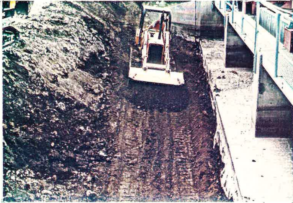
Photo No. 17 7-2-84 Gary McDowall, SWC Employee, Spreading Backfill Material With Our JD-555
