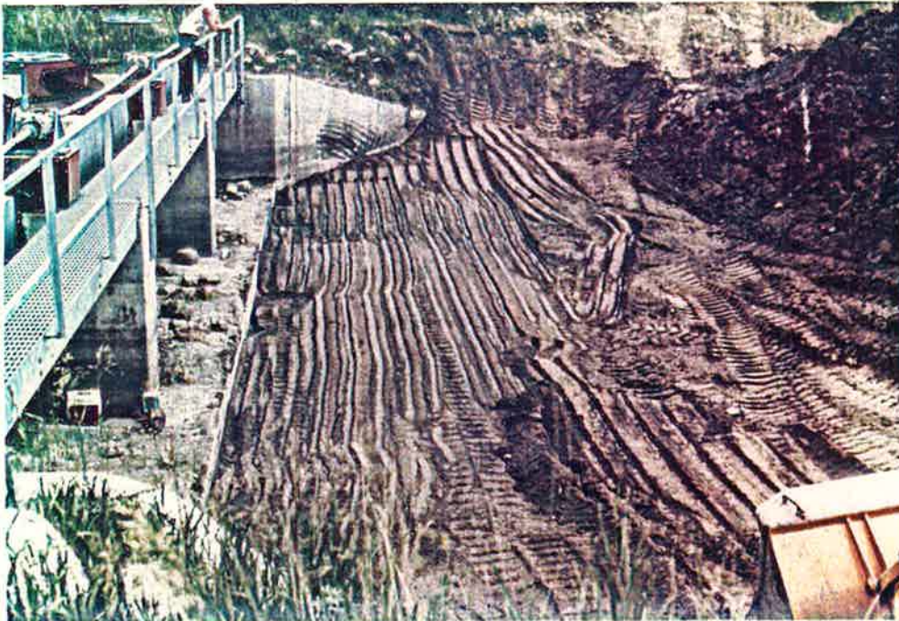
Photo No. 20 7-3-84 Placing the Sand-Gravel Filter Blanket
