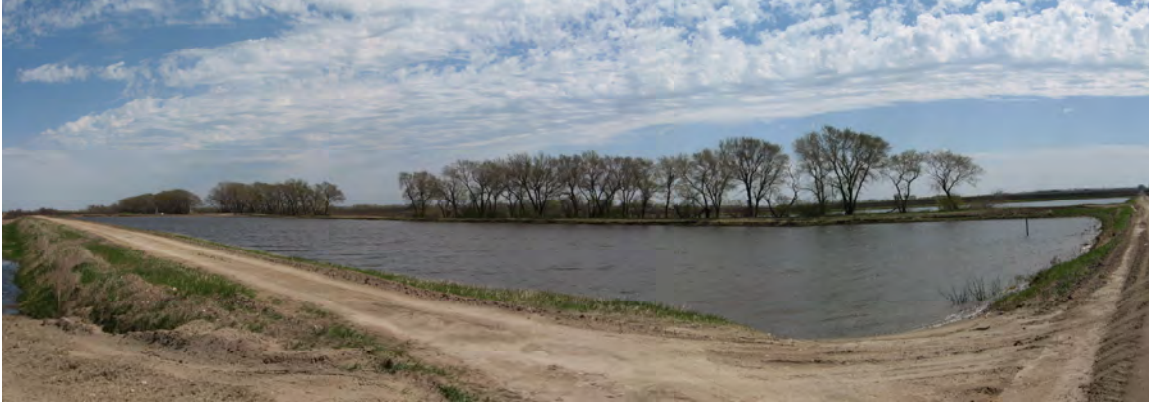
Figure 19. Aquifer recharge and recovery basin operated by the Forest River Hutterite Community to store and use high flows from the Forest River.
