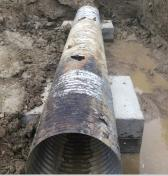
Before repairs were conducted, sagging and warping of the pipe and a sinkhole was forming. The pipe is shown with new supports after repairs were completed.
