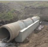
Prior to repairs, the footings for the pipe were deteriorating. After construction was finalized, the pipe was intact and reinforced.
