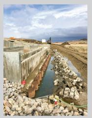
The Devils Lake East End Outlet, owned by the ND State Water Commission, discharges a maximum of 350 cubic feet per second of water from Devils Lake through an 8-foot diameter concrete pipe to an outfall structure in the Tolna Coulee five miles away. The outfall structure consists of a reinforced concrete spillway structure, an area of articulated concrete block for energy dissipation, and a sheet pile wall as the final stage.
