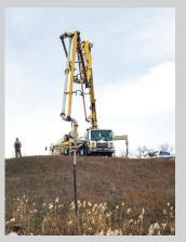
The State Water Commission construction crew filled the existing lowlevel conduits with a cement grout to seal them and eliminate the risk caused by the high-pressure water near the toe of the dam. In the spring of 2019, the plan is to install a new outlet conduit with control on the upstream side of the dam into the west embankment's principal spillway.
