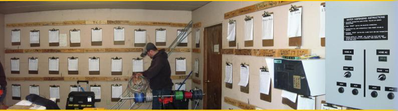
The city of Parshall's water depot during the installation of their new telemetry system in February 2012. The old billing system of 53 clipboards are still hanging on the walls. The new telemetry system is at the far right of the picture.
