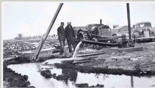
Pumping from a well on Turtle Lake in 1937. The first well project developed by the state water commission. Credit: ND Historical Society
