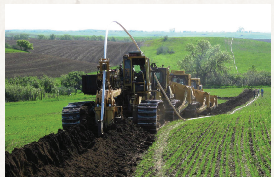
Water pipeline being installed, as part of SWPP.
