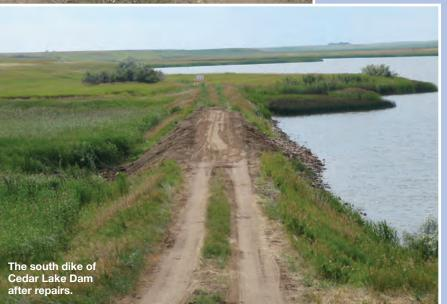
The NDGFD and the Slope County Water Resource Board (WRB) submitted a cooperative request to the Water Commission to assist with the needed repairs. As part of that process, the Commission's construction crew repaired the eroded areas with borrow from the adjacent landowner, who allowed access for the project. In addition, rock protection was also added on the upstream side of the south dike.
