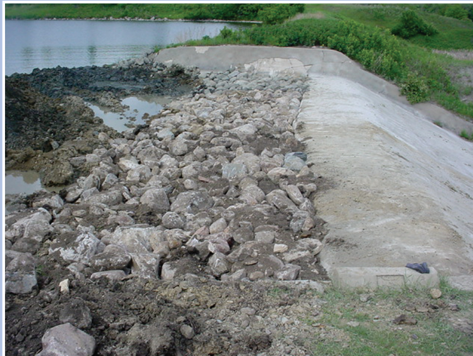
The newly repaired weir and rock-covered approach channel at Tolna Dam.
