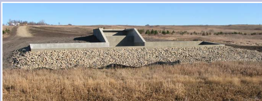
Terminal Structure: The terminal structure marks the end of the outlet, where water is discharged into the Sheyenne River. Construction on the outlet portion of the terminal structure is complete.
