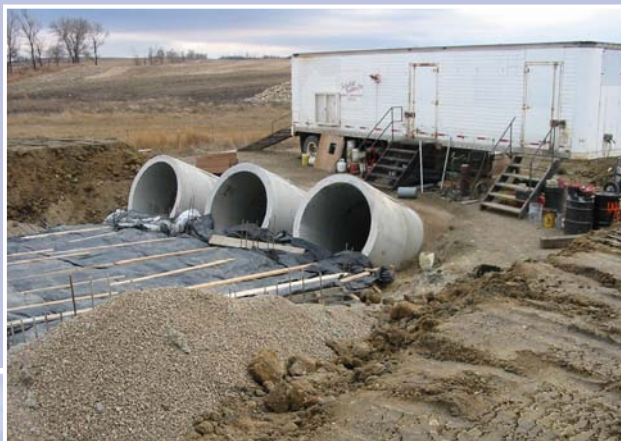
Siphons: A small amount of work remains on the siphon inlet and outlet structures, but all pipeline work has been completed. The siphons are constructed of three side-by-side 6-foot diameter reinforced concrete pipes.
