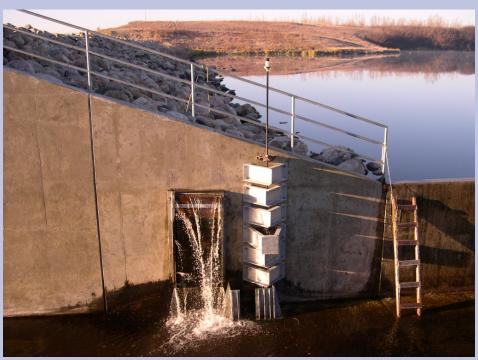
The stop-log structure that was installed in the Mount Carmel Dam spillway. Enough stoplogs can be removed to lower the reservoir up to 6 feet if necessary.
