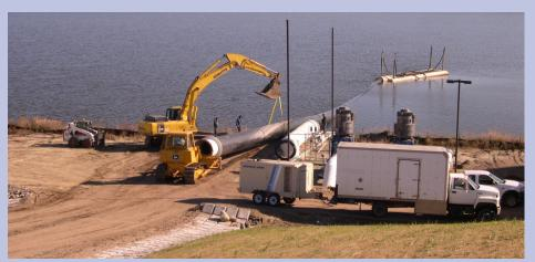
Removal of the Devils Lake Outlet Project intake pipe at the Round Lake pumping station.
