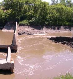
These two images show Colt Dam before its failure this past summer and after. The Water Commission's construction crew is currently in the process of removing the entire dam from the river channel.
