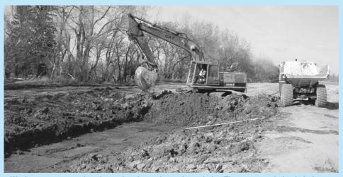
Workers are excavating the outlet channel near Long Lake. The excavated clay is being uses to line other sections of the Devils Lake Outlet channel.
