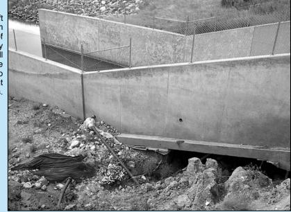
along with representatives from GEI participated in the site investigation. The Commission's survey crew was also present to obtain elevation data on the concrete chute spillway in order to determine the amount of movement of the structure.
