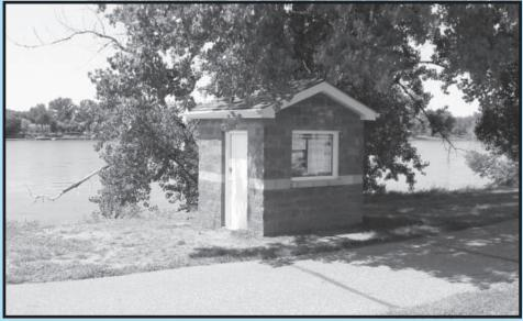
a change in the height of the river produces a corresponding change in the pressure in the pipe. This change then is converted to an electronic signal by a transducer inside the gage house. Data from the transducer is fed to a recorder, or data-collection platform, which records the corresponding river height.
