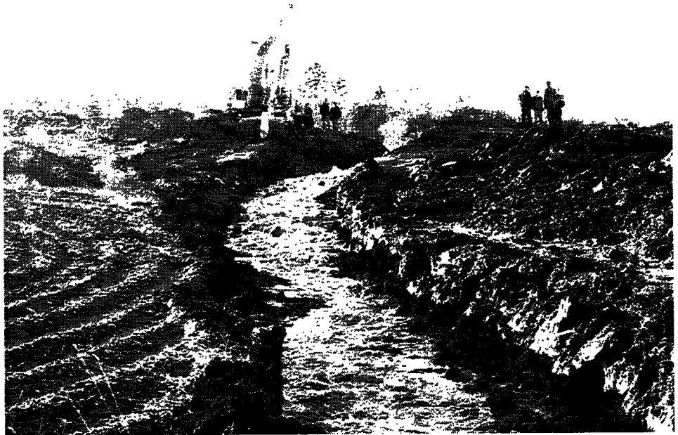
Emergency breach of Iverson Dam in Benson County.
