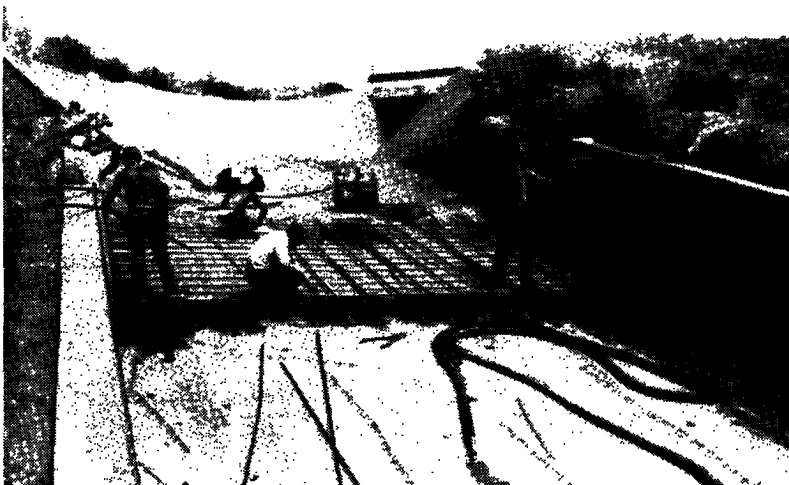
Epping Dam — Repair Work in Progress
