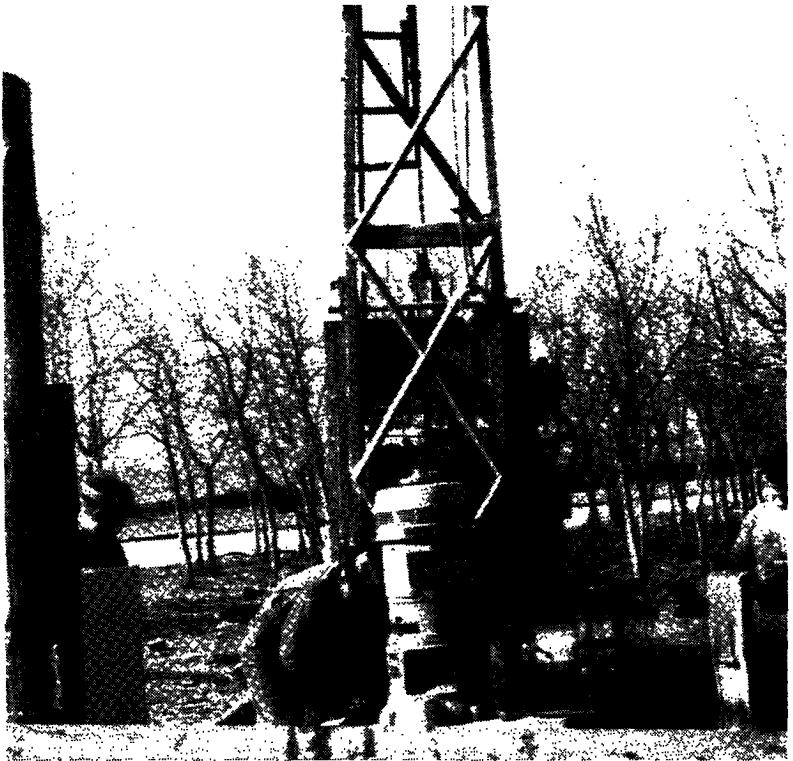
Cartwright Project Pump Installation
