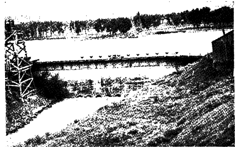
Intake Structure—Lower Yellowstone Project
