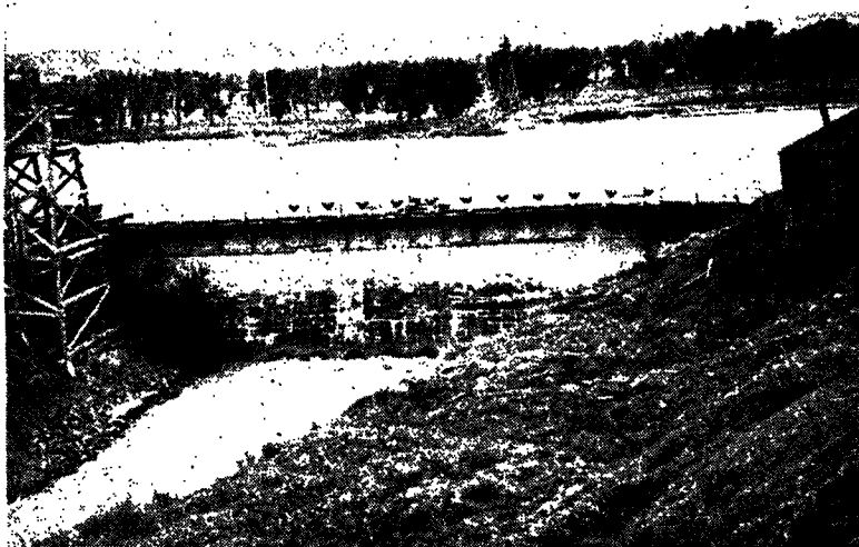
The diversion dam and intake structure near Savage, Montana, on the Lower Yellowstone Project. The project canal is in the foreground and the dam may be noted by the riffle extending across the river between the two towers.
