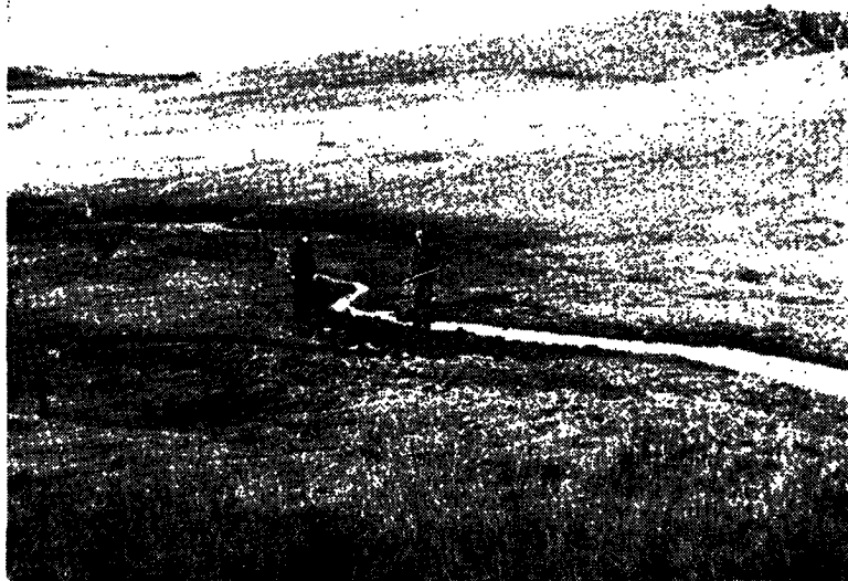
Diverting waters from a coulee over a flat meadow located at the foot of the hills. Note small earth barrier in front of men, which has diverted stream from its original channel so the water may flow along toe of hill and spread over meadow.
