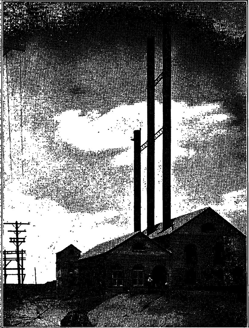
POWER HOUSE FOR WILLISTON AND BUFORD-TRENTON PROJECTS.
